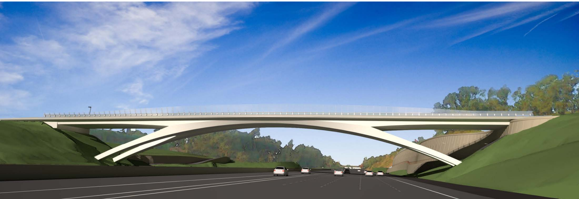
Gilman Bridge Northbound Elevation
