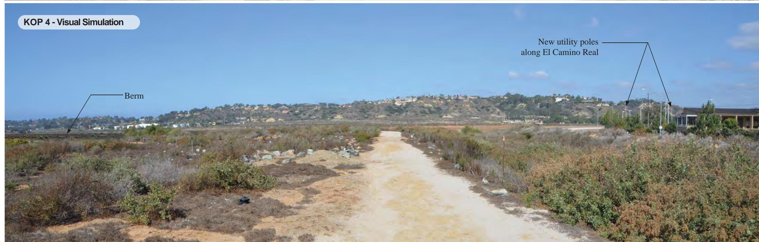
Note: The new (temporary) poles along El Camino Real are required if undergrounding does not occur prior to this project. It may be possible to relocate 2 existing electrical lines (12Kv : 69Kv) on existing structures within current utility corridor instead of relocating existing poles. This represents worst-case pole configuration.
