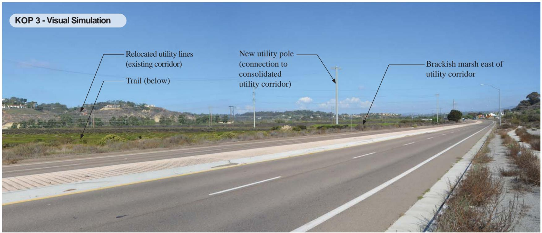
Note: The new (temporary) poles along El Camino Real are required if undergrounding does not occur prior to this project. It may be possible to relocate 2 existing electrical lines (12Kv : 69Kv) on existing structures within current utility corridor instead of relocating existing poles. This represents worst-case pole configuration.
