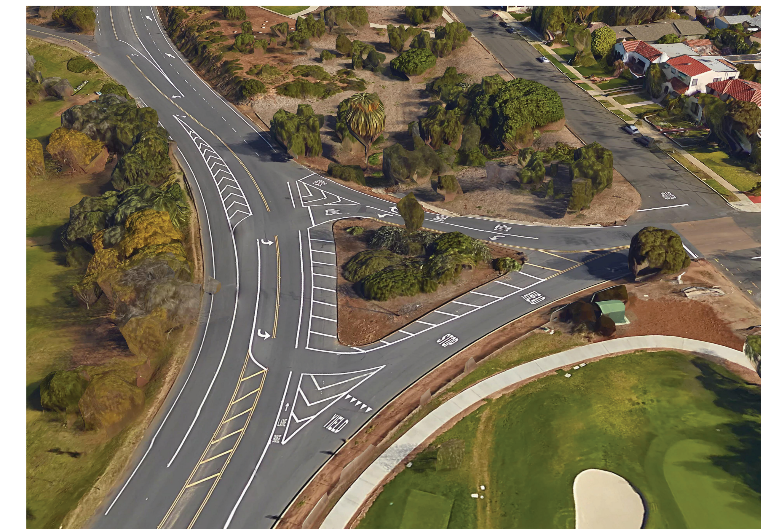
There is currently no safe crossing option from 28th Street to Florida Drive within Balboa Park. Introducing a roundabout to this intersection will enhance safety and connectivity.
