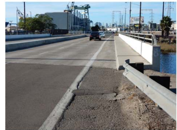
Chollas Creek bridge, looking north.
