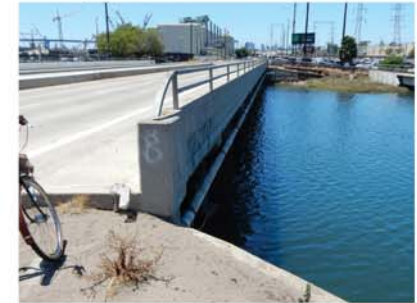
North side of Chollas Creek bridge.
