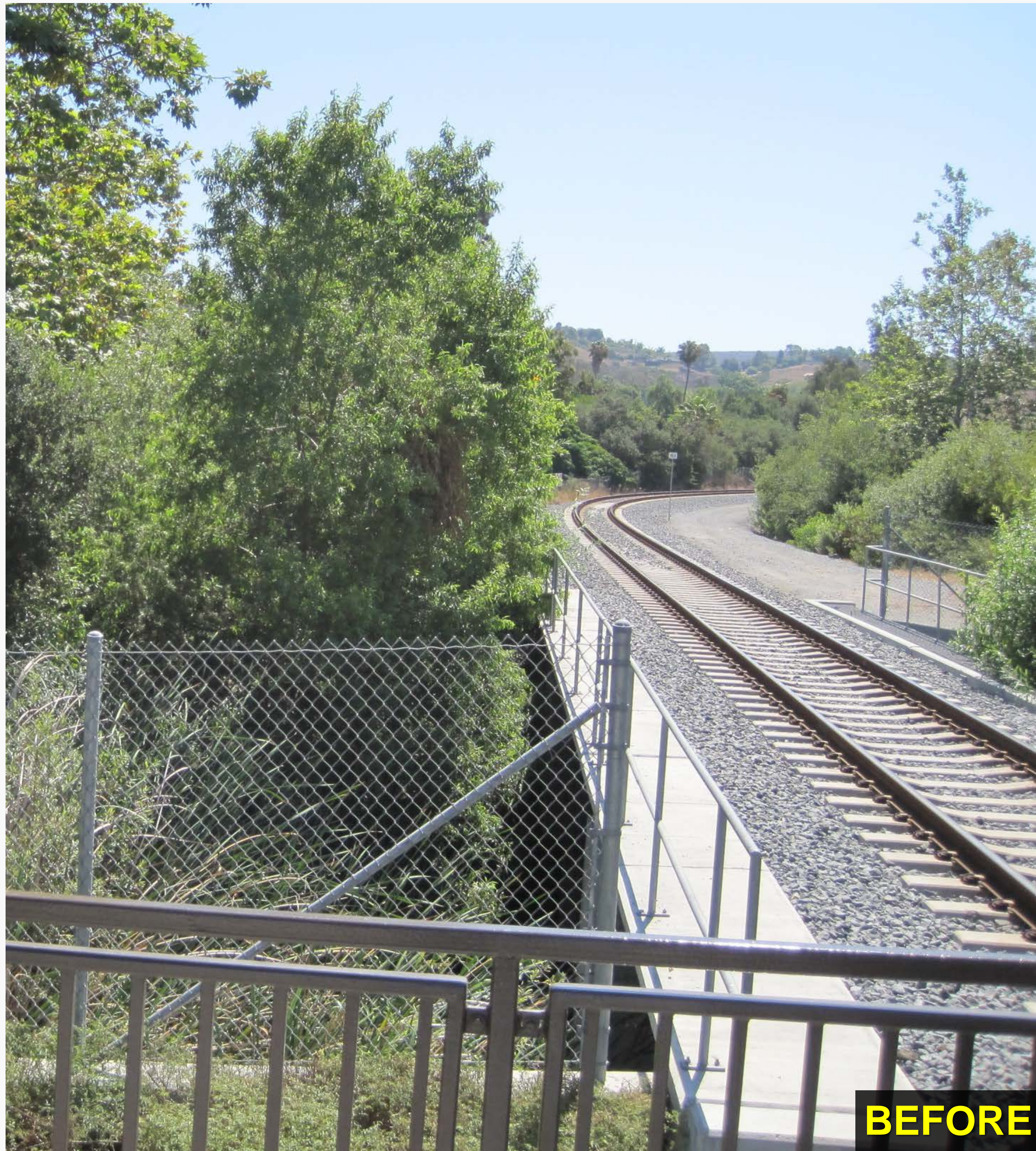
Key view looking east from Buena Creek Transit Station
