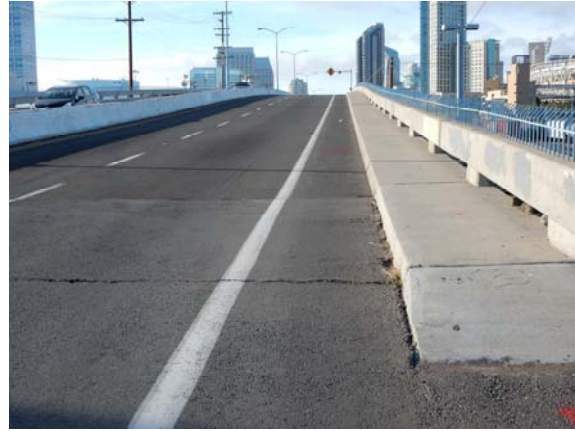
Figure 23: View north on Harbor Drive Bridge near Tenth Avenue Marine Terminal
