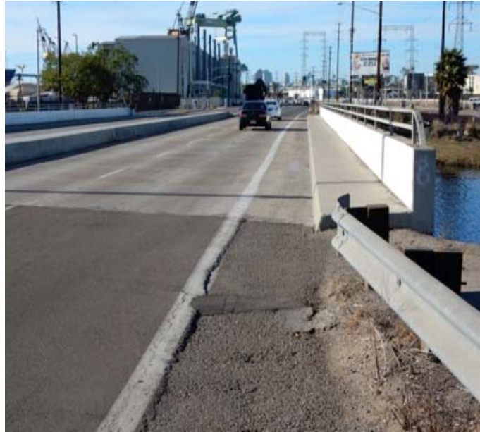
Figure 16 - Chollas Creek Bridge - potential bikeway alignment
