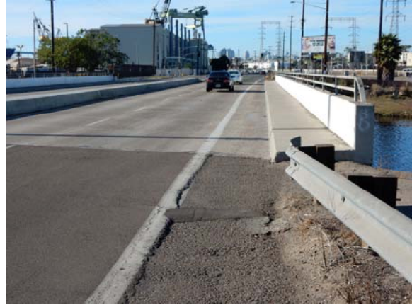
Figure 27: Chollas Creek Bridge
