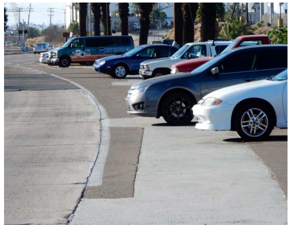
Figure 15 - Vehicles west of 28th St encroaching on existing bike lane
