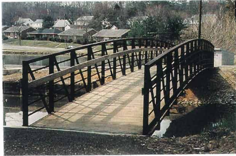
Pedestrian bridge - Fredericksburg, Virginia
