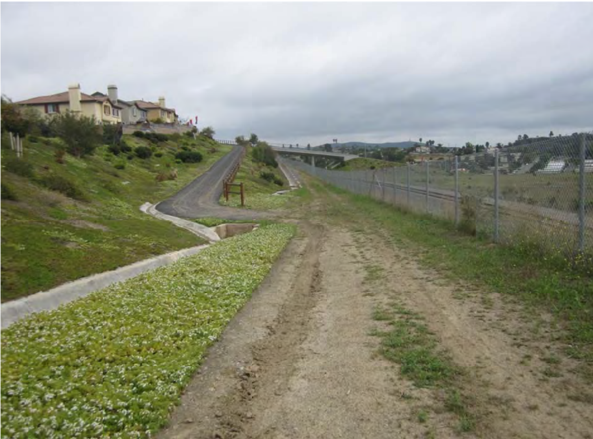
Photograph 4. Representative landscaping associated with the housing development east of Santa Fe Avenue.
