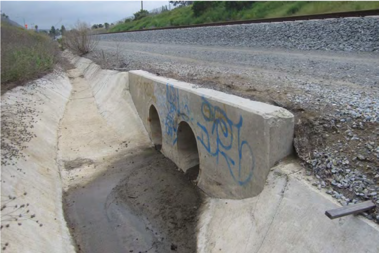
Photograph 12. Representative concrete lined drainages within the NCTD ROW.
