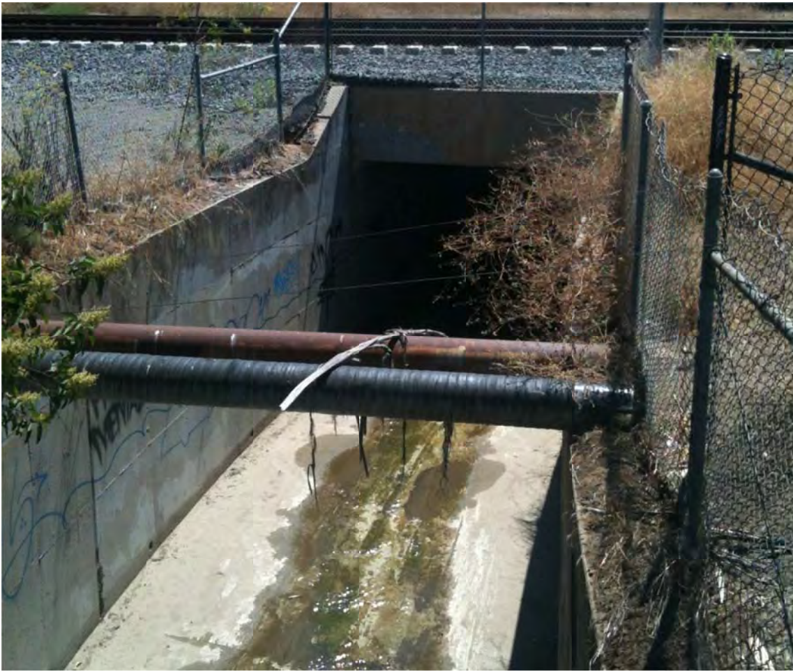
Photograph 11. Representative concrete lined Buena Vista Creek.
