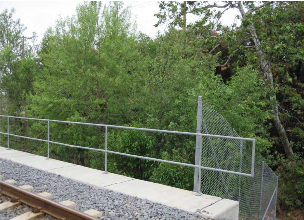
Photograph 5. Representative Southwestern Willow Riparian Forest vegetation north of the NCTD rail Buena Creek crossing.
