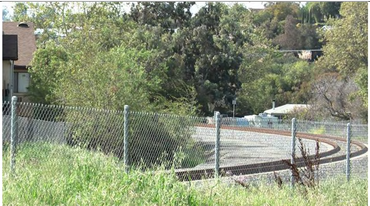
Photo 3b. WP 315: Looking west. Willows on south side of track extending east along housing but adjoining Buena Creek which runs north/south where it crosses the track at Buena Creek Station.
