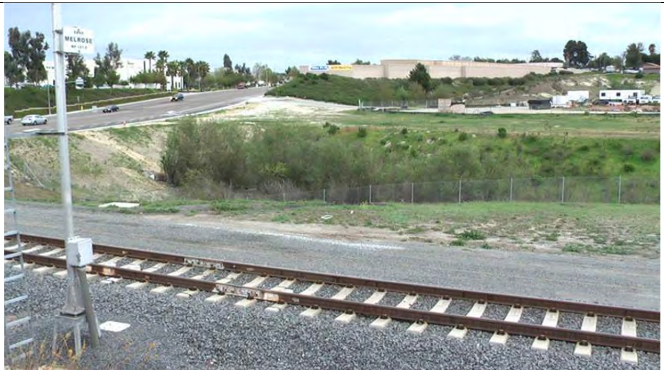
Photo 7. WP 326: Looking south from Melrose Station at willow riparian restoration project south of ROW fence with NNG on either side of the drainage.
