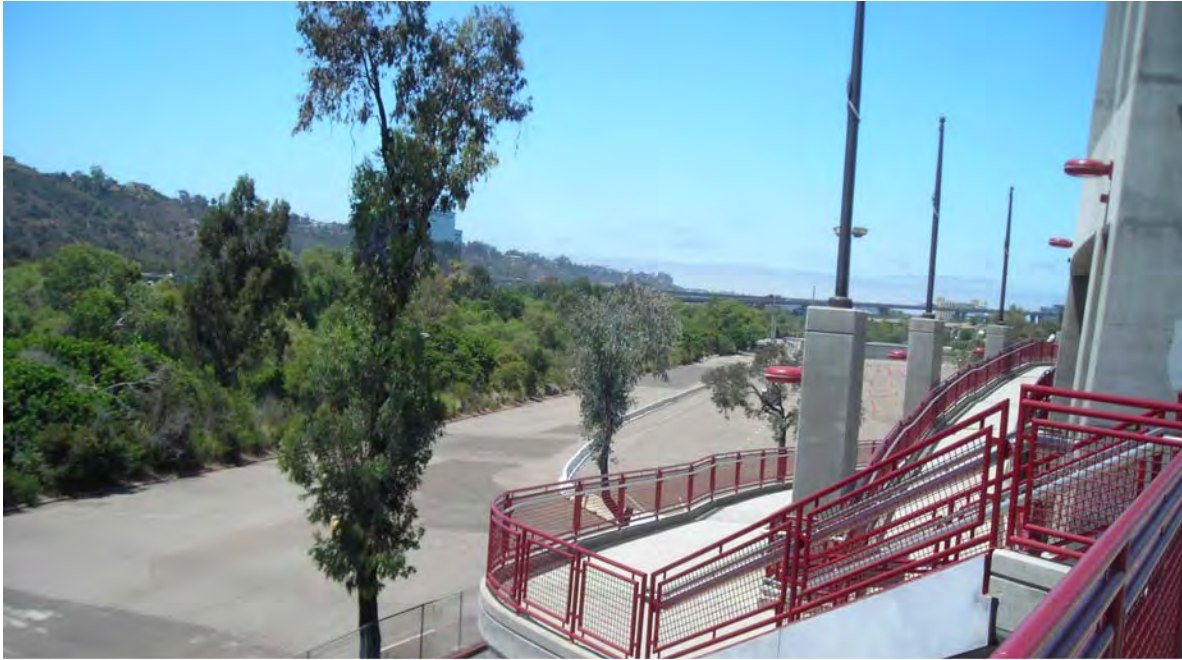
View looking west along the proposed project alignment from the Qualcomm Trolley Station.
