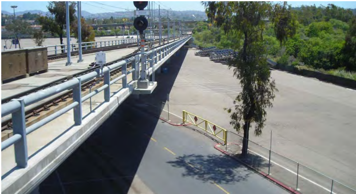
View looking east along the proposed project alignment from the Qualcomm Trolley Station. The bleacher storage area is visible on the photograph.
