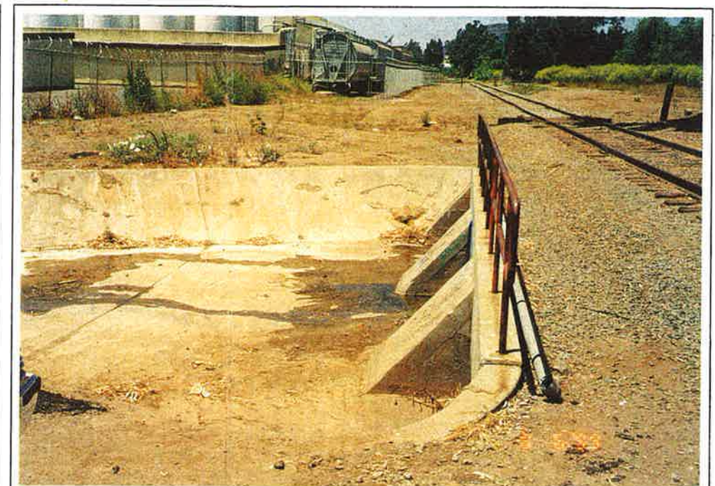
o: northwest-facing view of typical span bridge crossing location.
