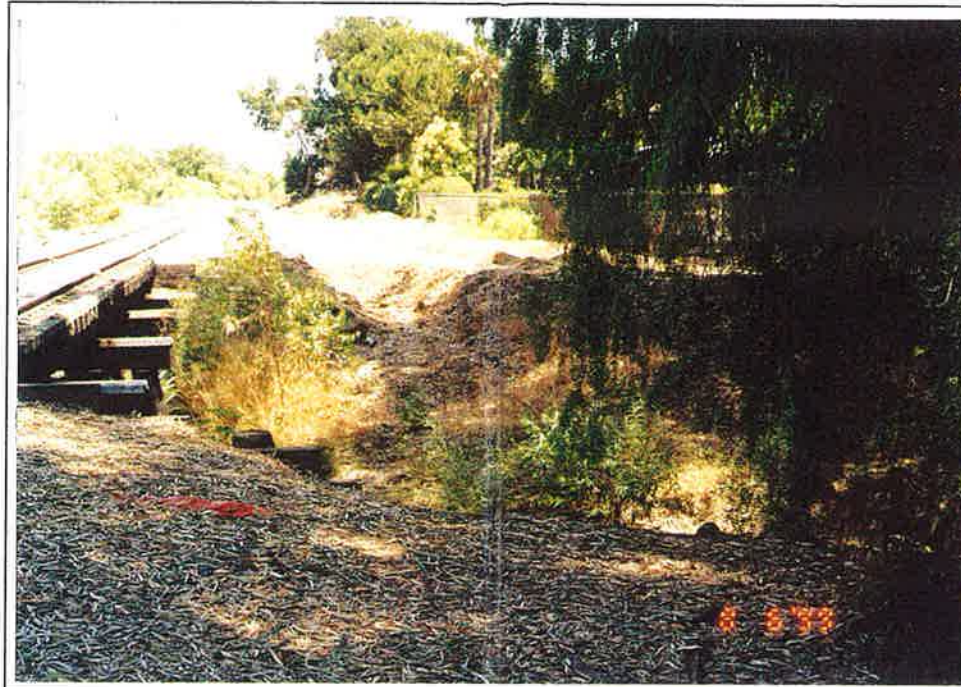
n: East-facing view of span bridge crossing location.
