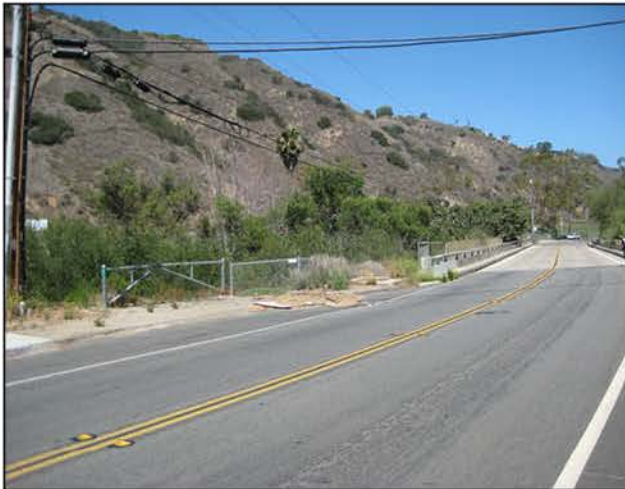
Photograph 9: Santa Fe Drive bridge over Rose Creek, looking northward
