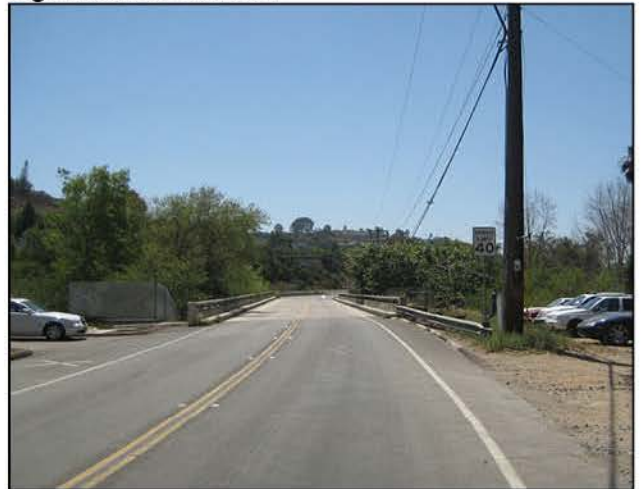
Photograph 10: Santa Fe Drive bridge over Rose Creek, looking southward
