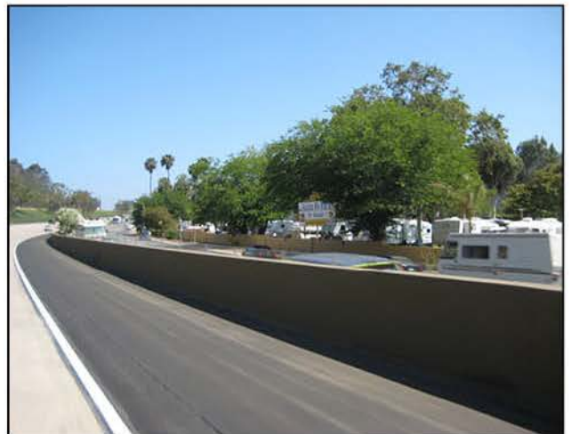
Photograph 12: View eastward from northbound I-5
