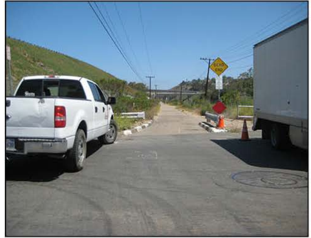
Photograph 14: Northward view at the end of Santa Fe Street/connection to existing Rose Creek Bike Path
