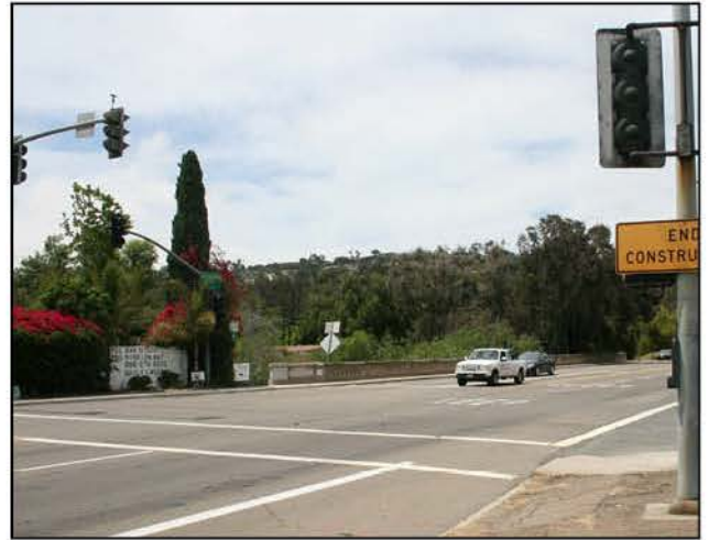
Photograph 2: Mission Bay Drive overcrossing over Rose Creek looking westward from Damon Street
