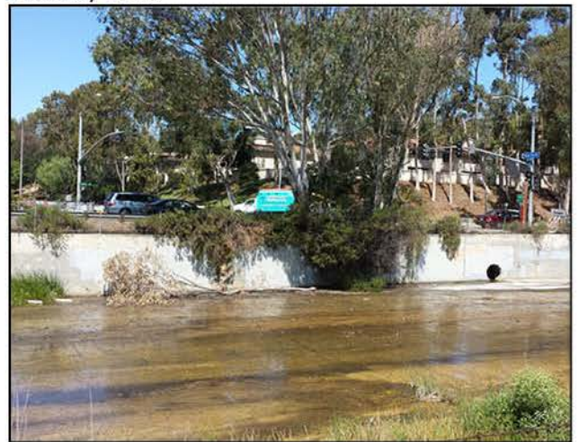
Photograph 6: Northwestward view of residential units near Mission Bay Drive and Bluffside Avenue
