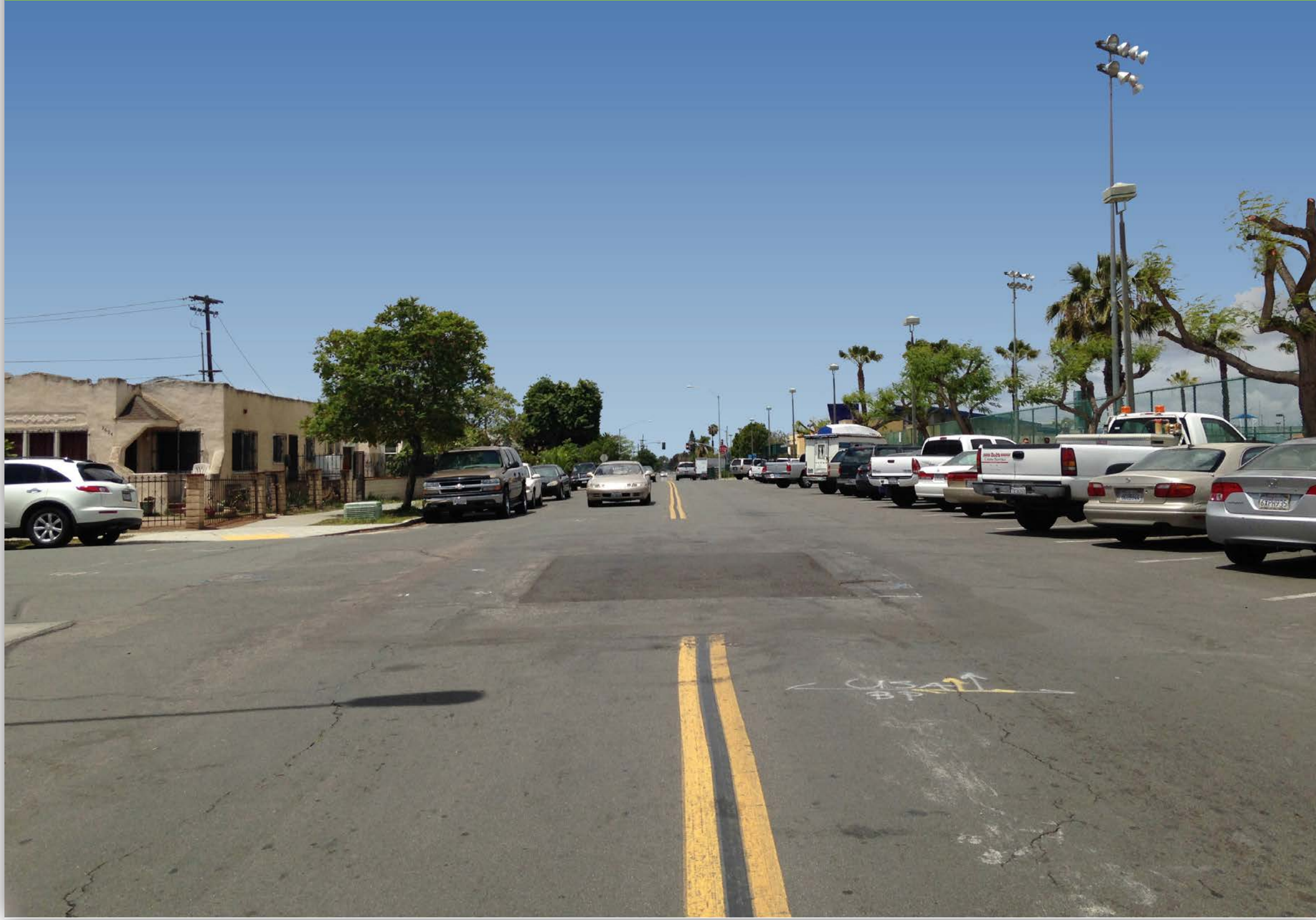
Landis and Highland - Before
