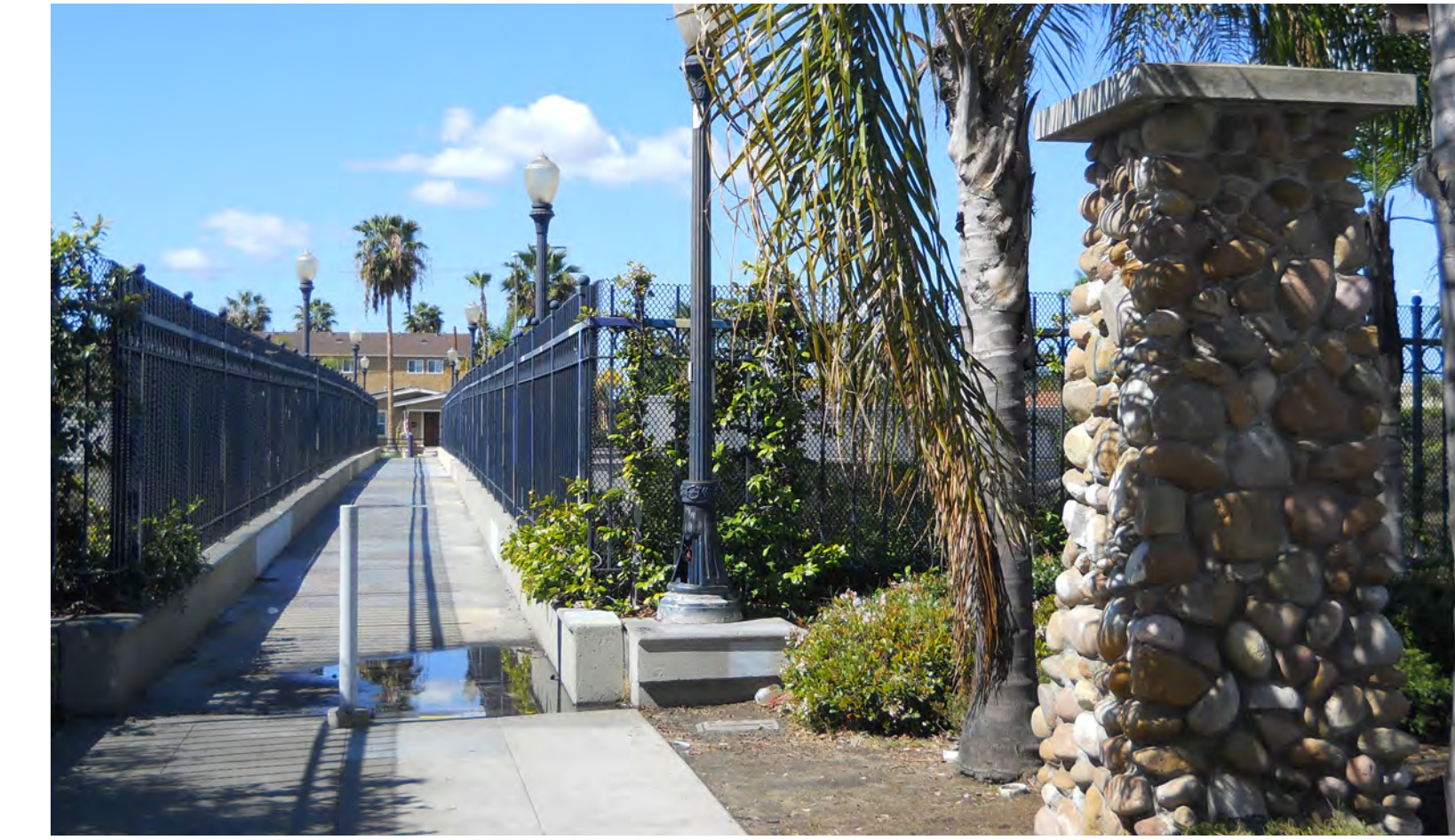
MONROE AVENUE PEDESTRIAN BRIDGE
