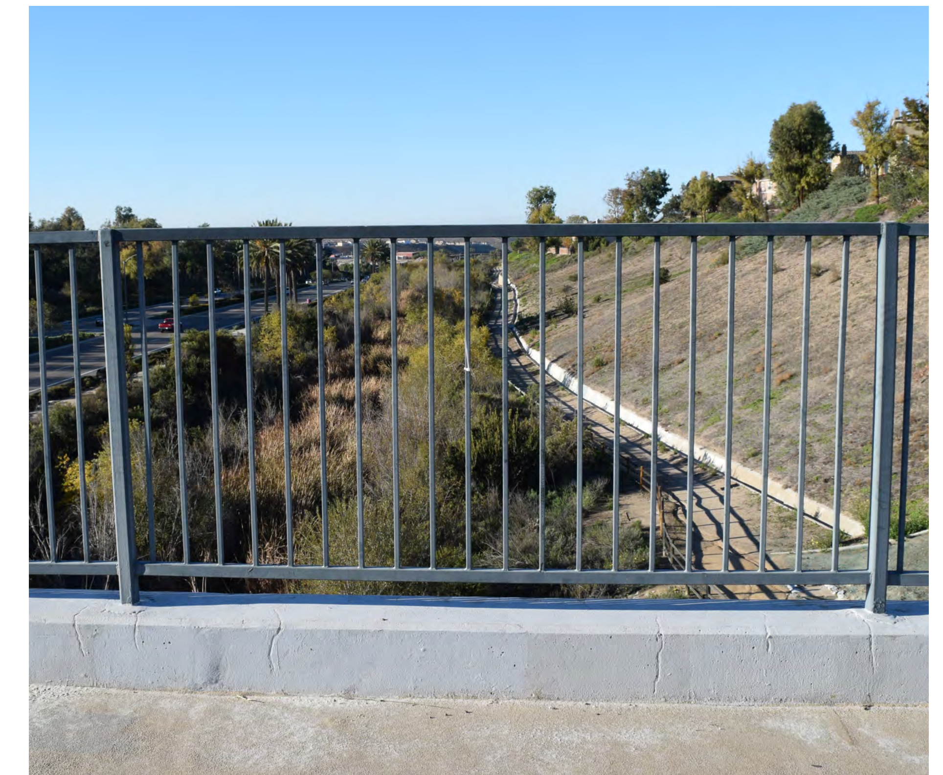
CHULA VISTA PEDESTRIAN BRIDGE
