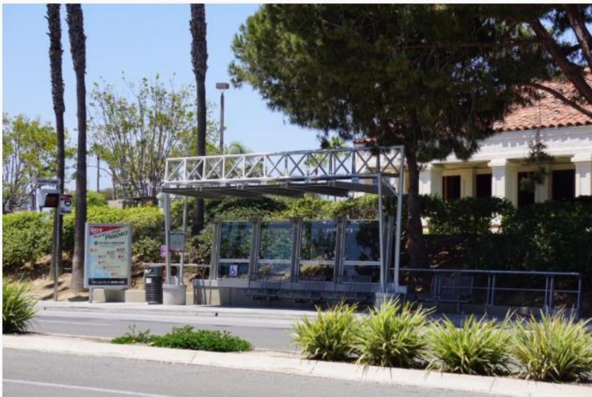
SANDAG's SuperLoop Rapid Station in University City. Photo courtesy of SANDAG
