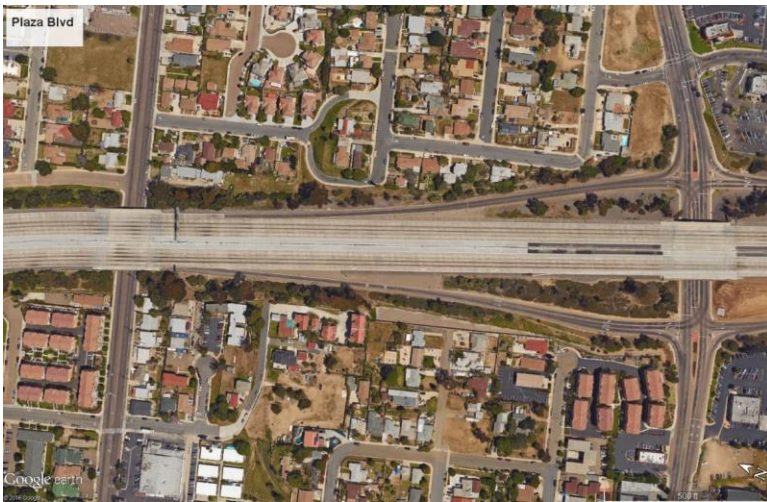
Plaza Blvd Interchange NB On/SB Off
