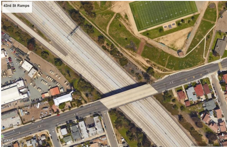
43 rd St Interchange SB On/NB Off
