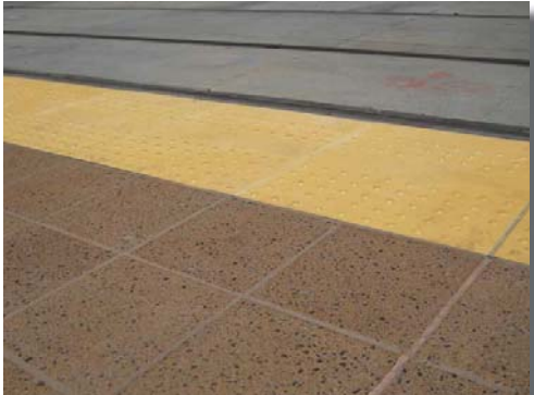
PLATFORM EDGE AND YELLOW TACTILE DOME
