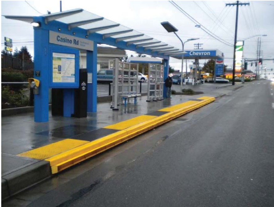
Community Transit – Snohomish County, Washington (Near-Level Boarding with 10-inch Curb)
