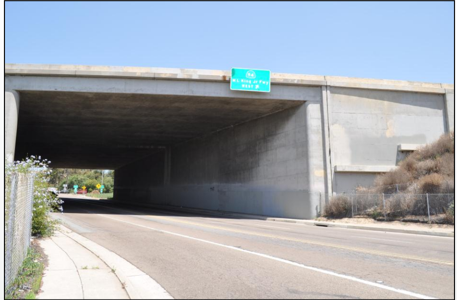
SR 94 at 32 nd Street
