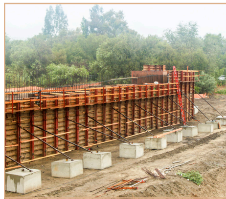
Framing the west side of the bridge’s base.
