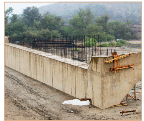
Building the east side of the bridge’s base.
