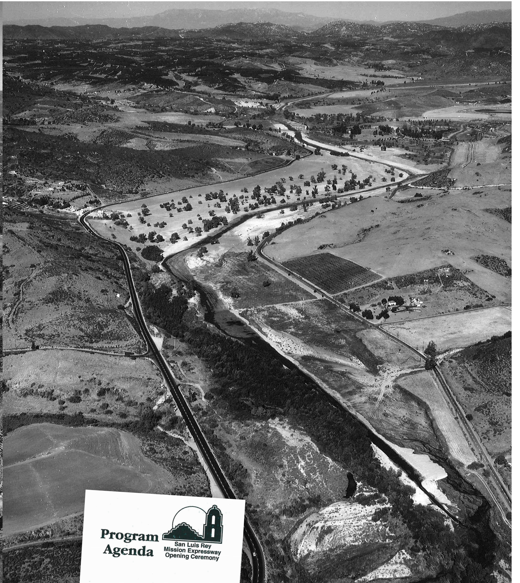
Looking East, State Route 76
