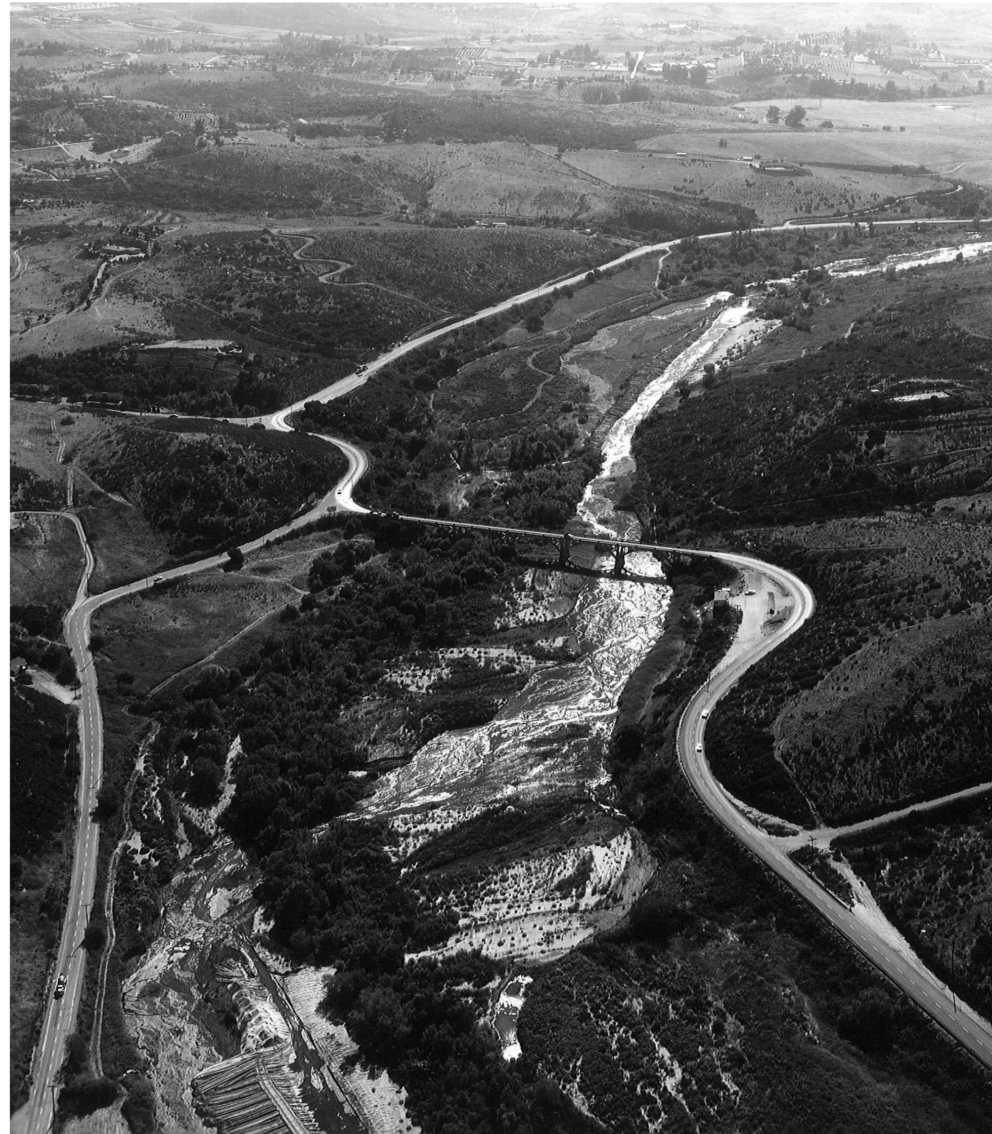
Looking West, San Luis Rey River Bridge
