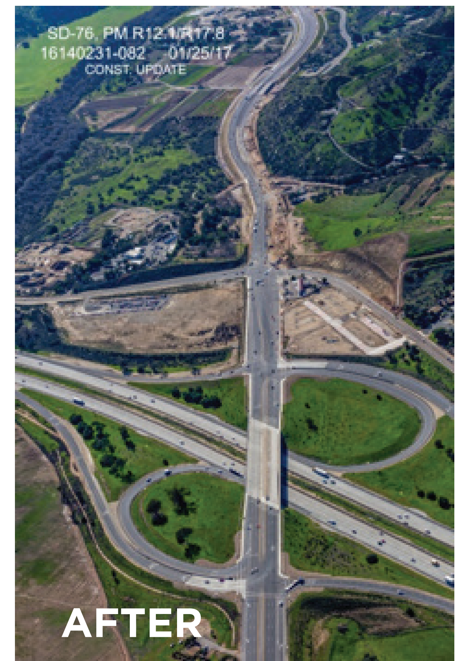
SR 76/I-15 Interchange
