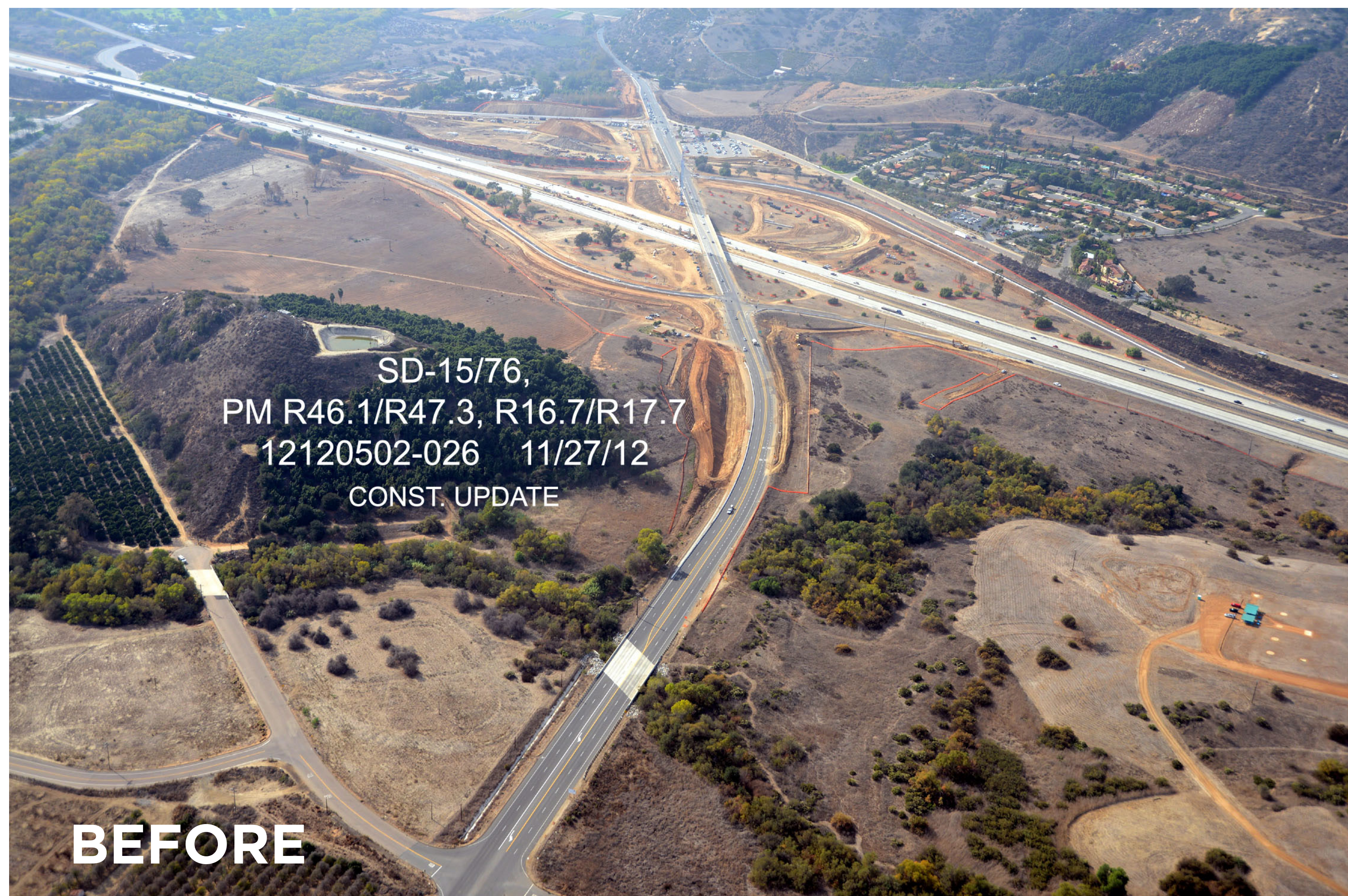
SR 76/I-15 Interchange
