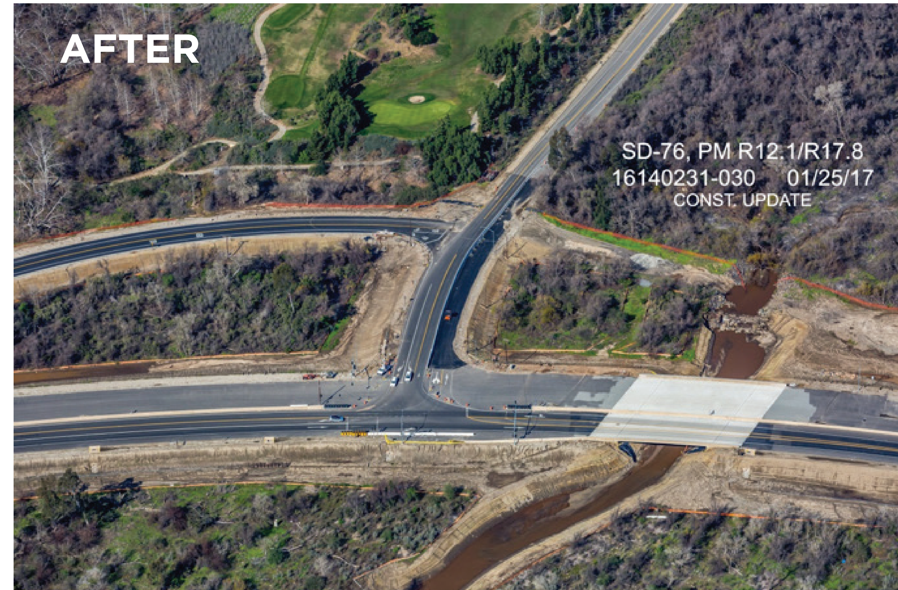
Intersection of Gird Road and SR 76
