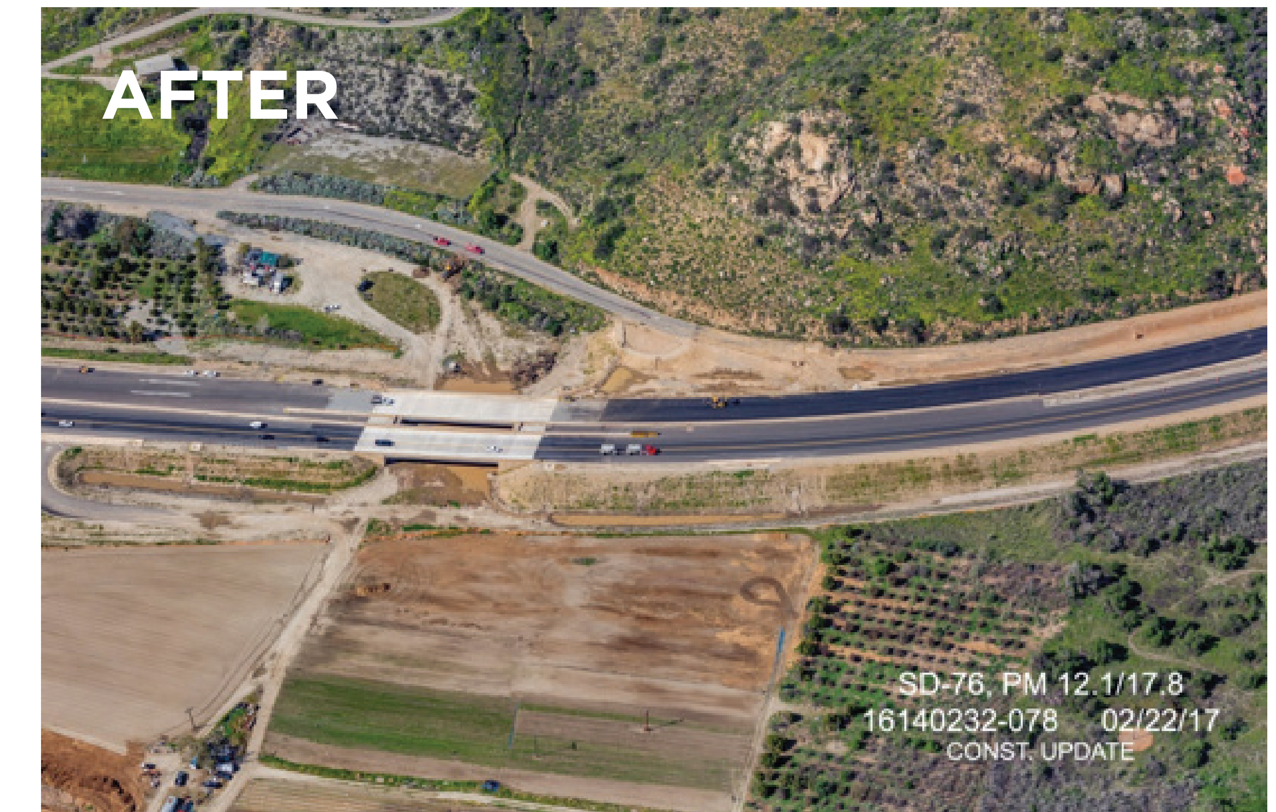
San Diego County Water Authority bridge
