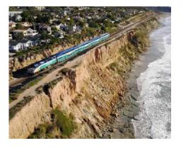
seismic events. Directing stormwater runoff more effectively across the bluffs will help lower the potential for erosion during large storm events. The installation of support columns will further help to protect the track bed from erosion and earthquakes.
