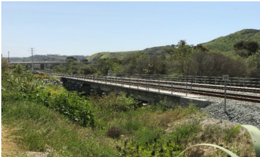
Figure 3 - SVDT Bridge 248.7 Post-Project Photo
