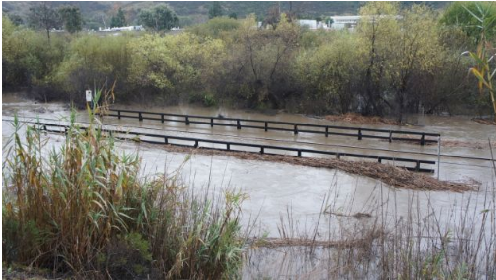
Figure 2 - SVDT Bridge 248.7 Pre-Project Flooding Photo
