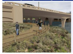
The San Elijo Lagoon highway bridge will be replaced to accommodate new Carpool/HOV Lanes along I-5. The new bridge will be lengthened to improve tidal flows, circulation, and the overall health of the lagoon. In addition, Caltrans will divert highway runoff into natural treatment features such as bioswales and detention basins to prevent runoff from entering the lagoon.
