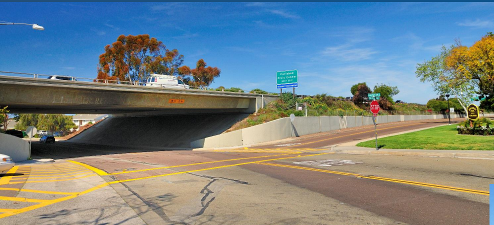
Existing Chestnut Avenue Undercrossing at I-5
