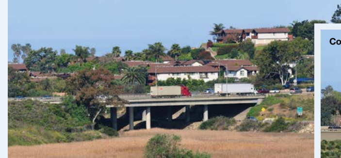
Existing Condition: I-5 North near Manchester Avenue
