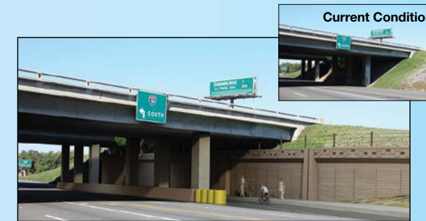
A new highway undercrossing at Encinitas Boulevard will include sidewalks and bike lanes, providing better east-west connectivity.
