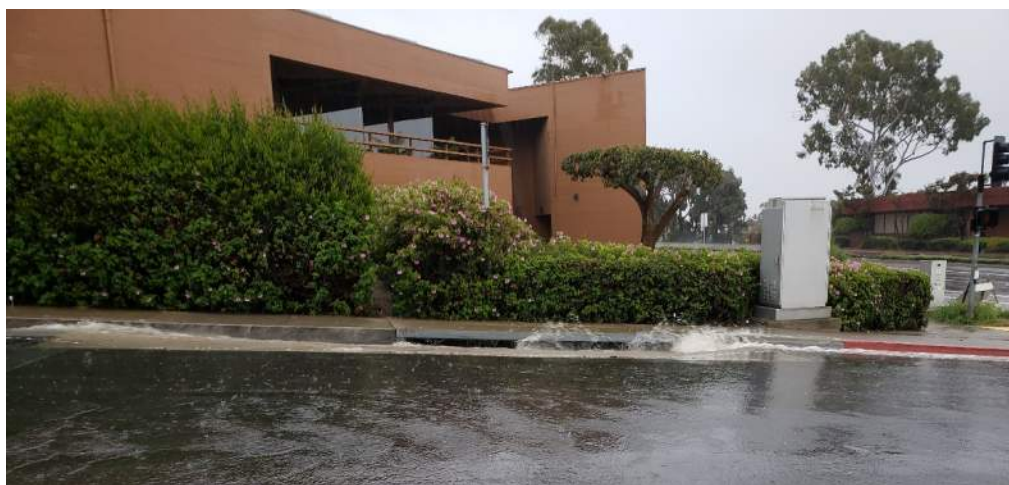
Figure 4. 9 th Street – Inlet Bypass
