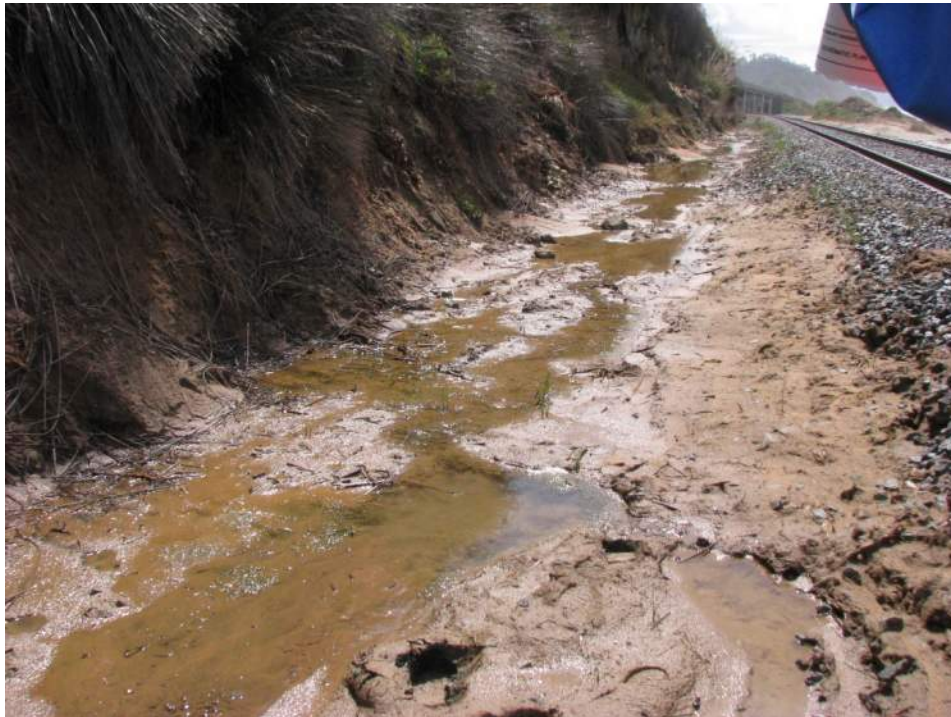
Figure 6. Existing Trackside Channel South of Anderson Canyon
