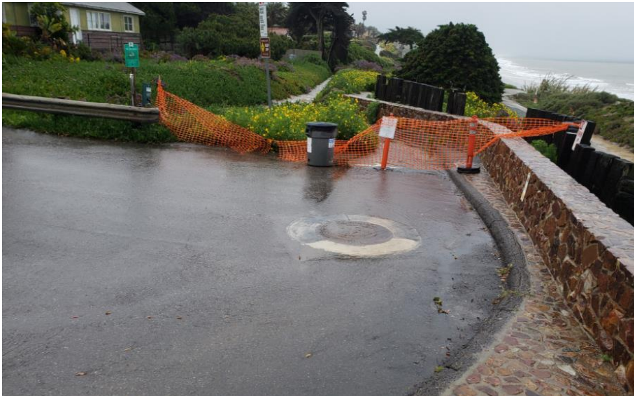
Figure 33 – Photo of Existing Rockwall at 9 th Street
