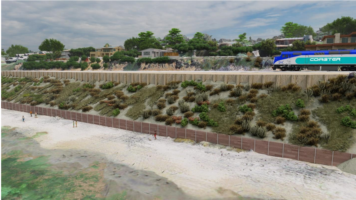
Figure 46 – Construction of improvements at the bluff top in conjunction with bluff toe and bluff face stabilization
