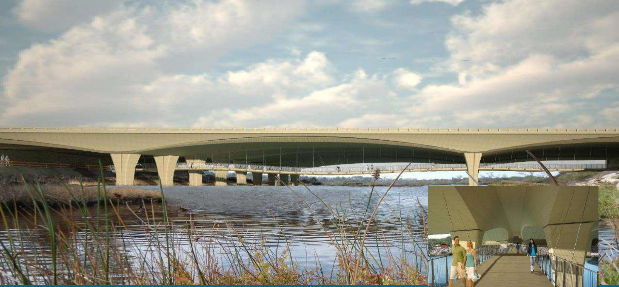
Visual simulation of the final San Elijo Lagoon Highway Bridge with suspended bike/pedestrian bridge
