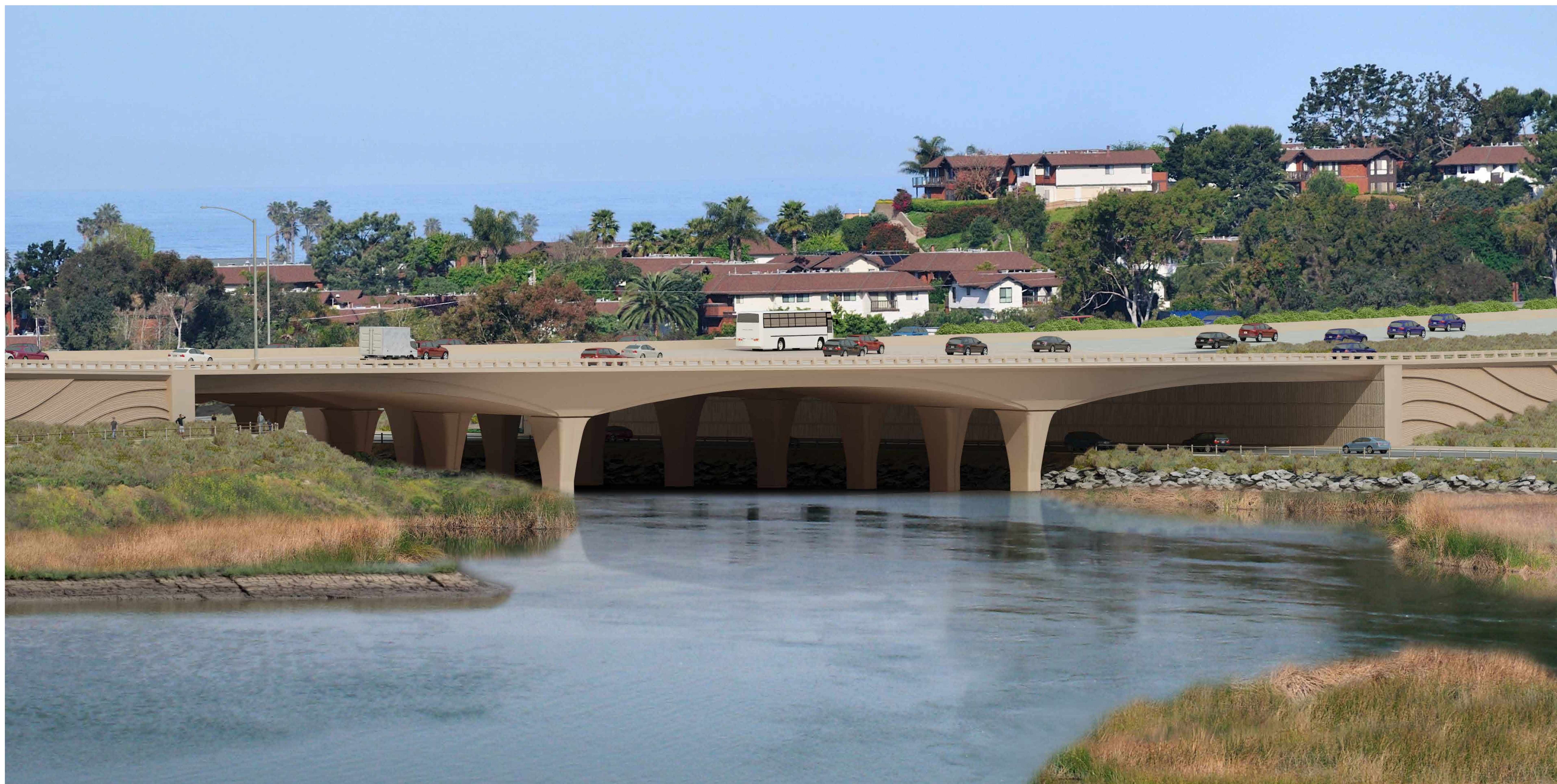
View looking northwest towards I-5 highway bridge over the San Elijo Lagoon and Manchester Avenue in Encinitas
