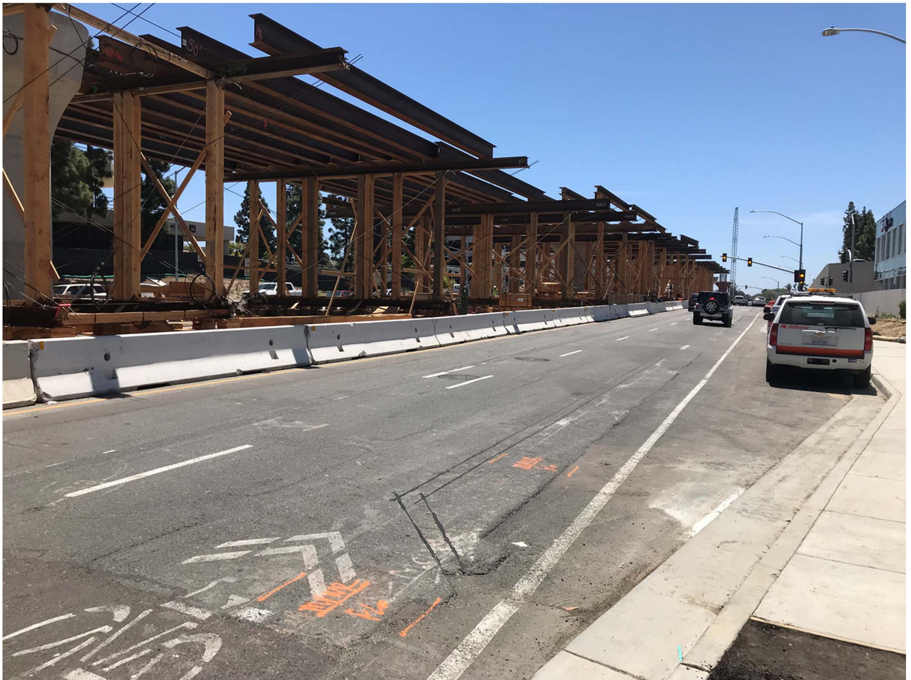
Falsework for the Executive Drive Station (looking south on Genesee Ave)
