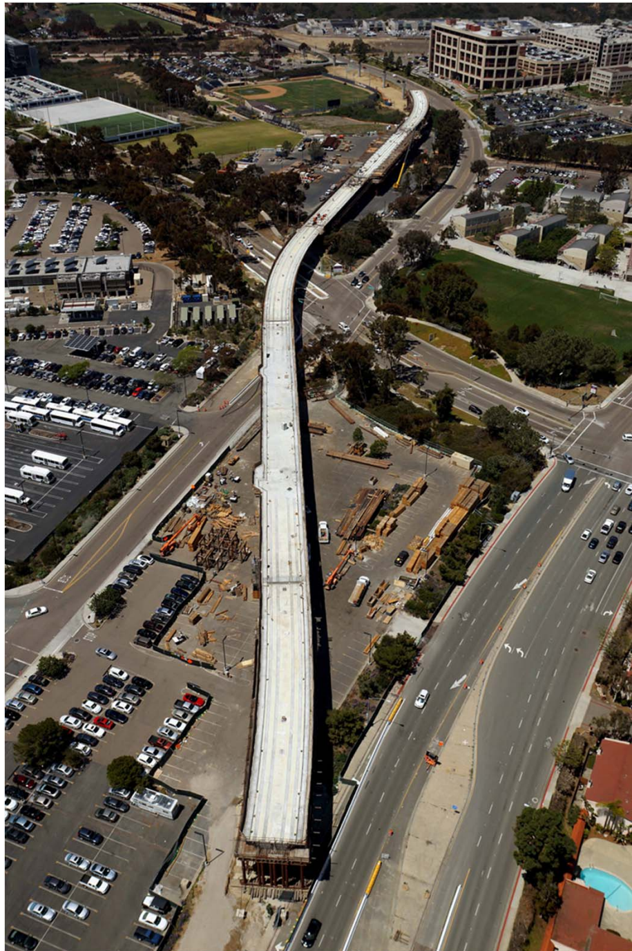
Looking west at UCSD Viaduct with Genesee Ave in foreground
