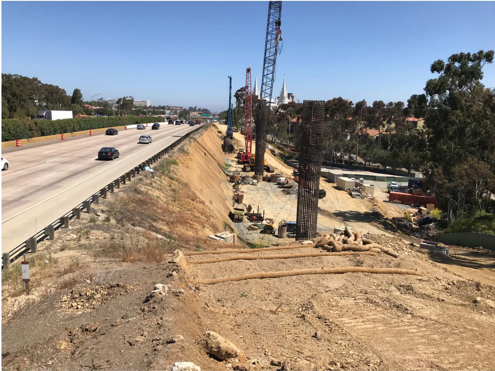
Looking North at Nobel Viaduct
