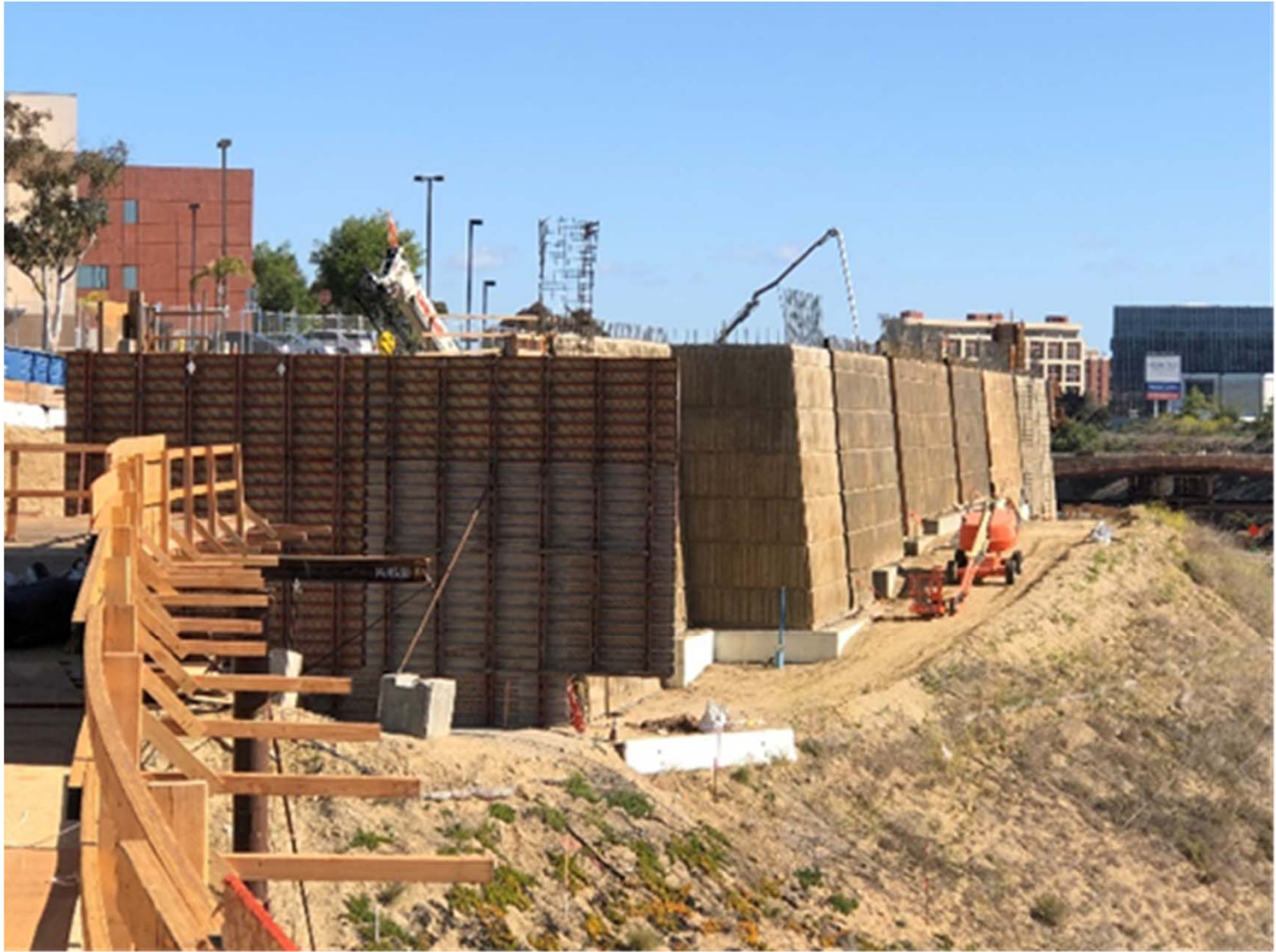
Progress at the VA Medical Center Station (Retaining Wall 848)
