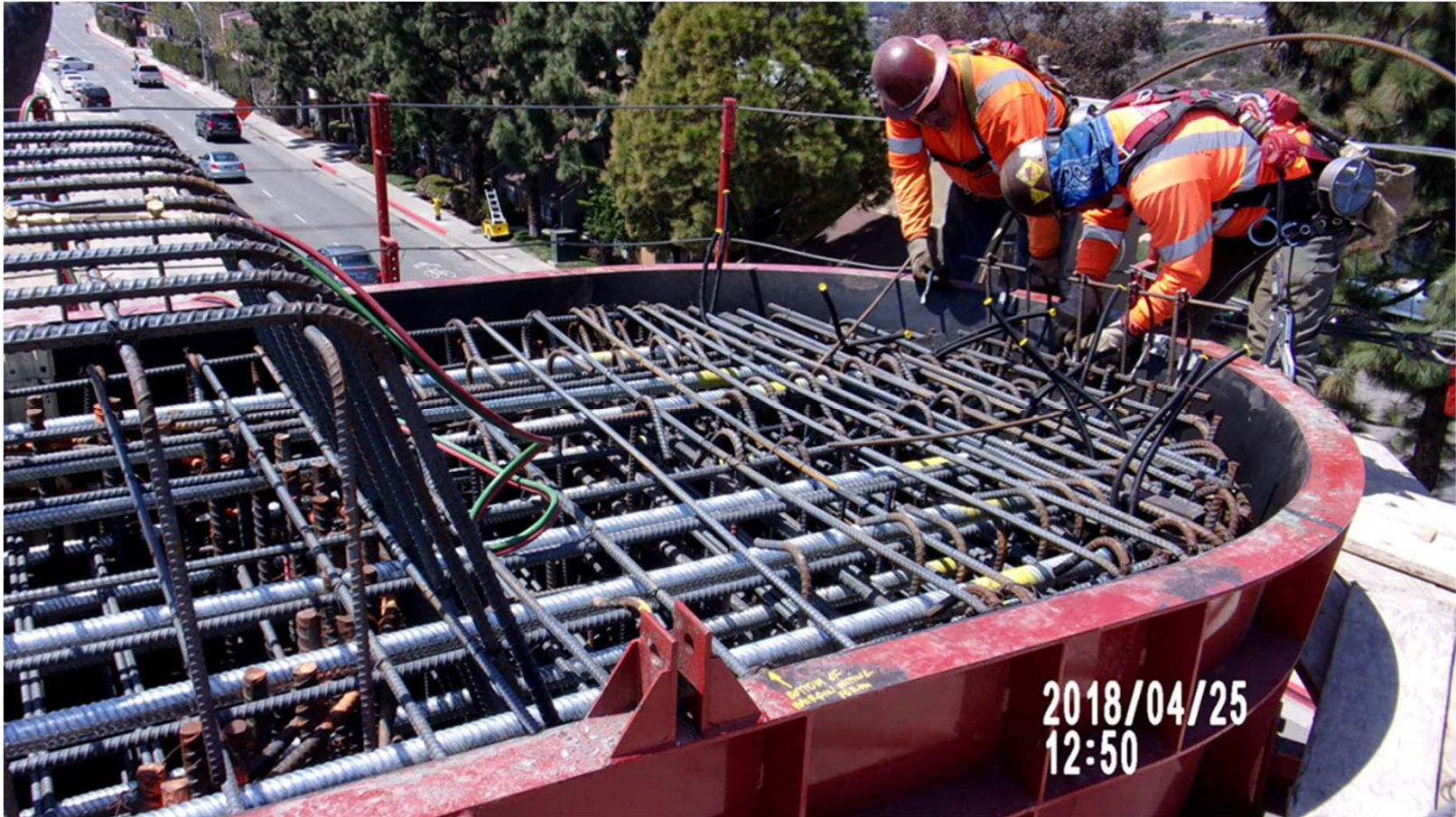
Completing upper column flare rebar cage at Genesee Viaduct Bent # 4
