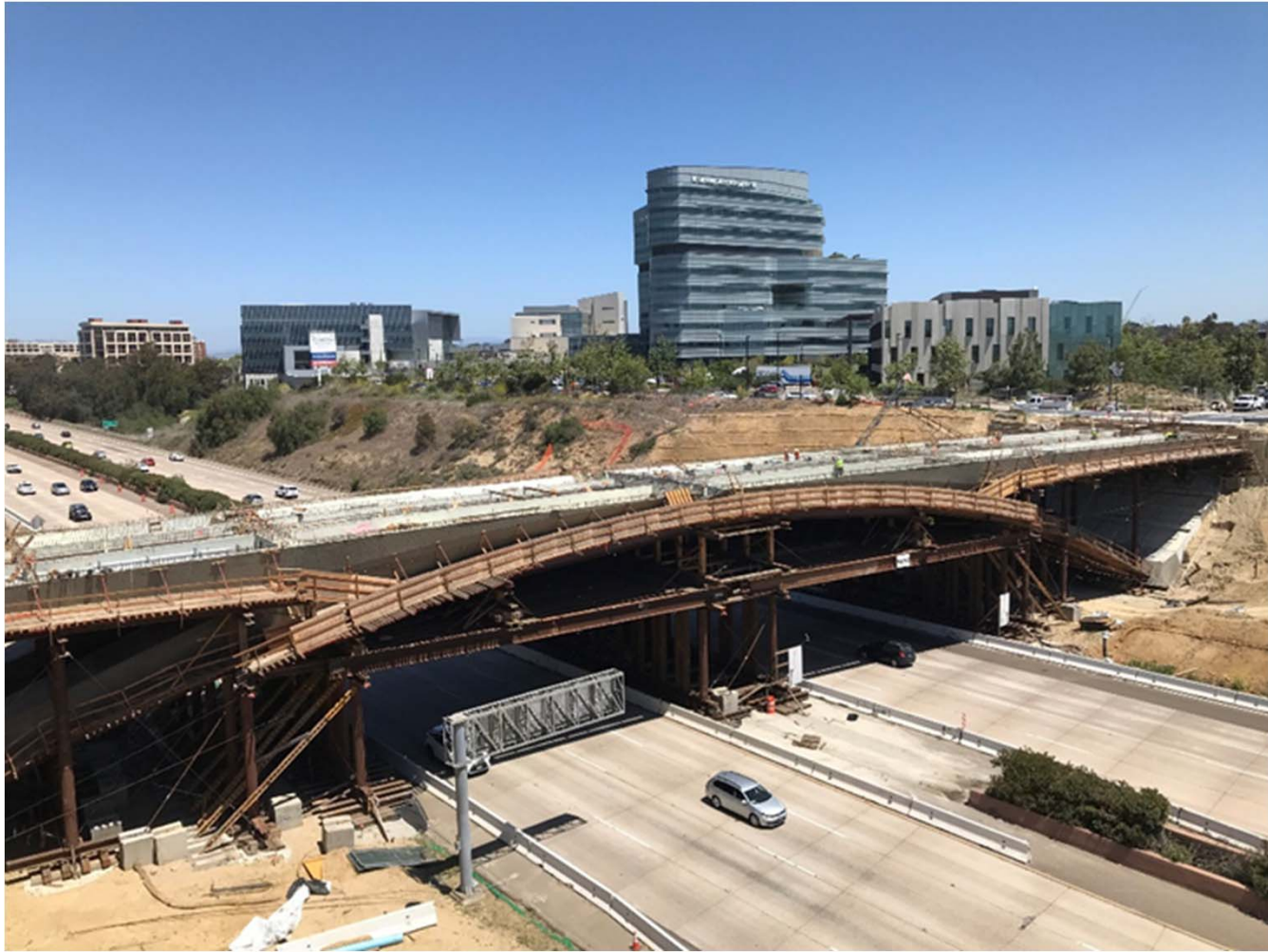
Gilman Bridge, looking northeast
