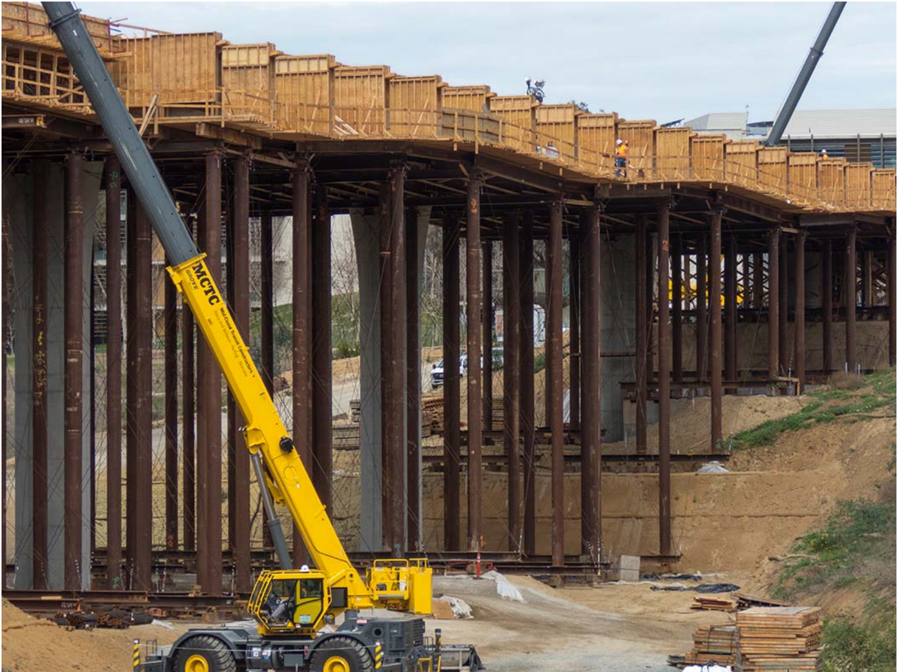
Pepper Canyon / UCSD West Station Falsework
