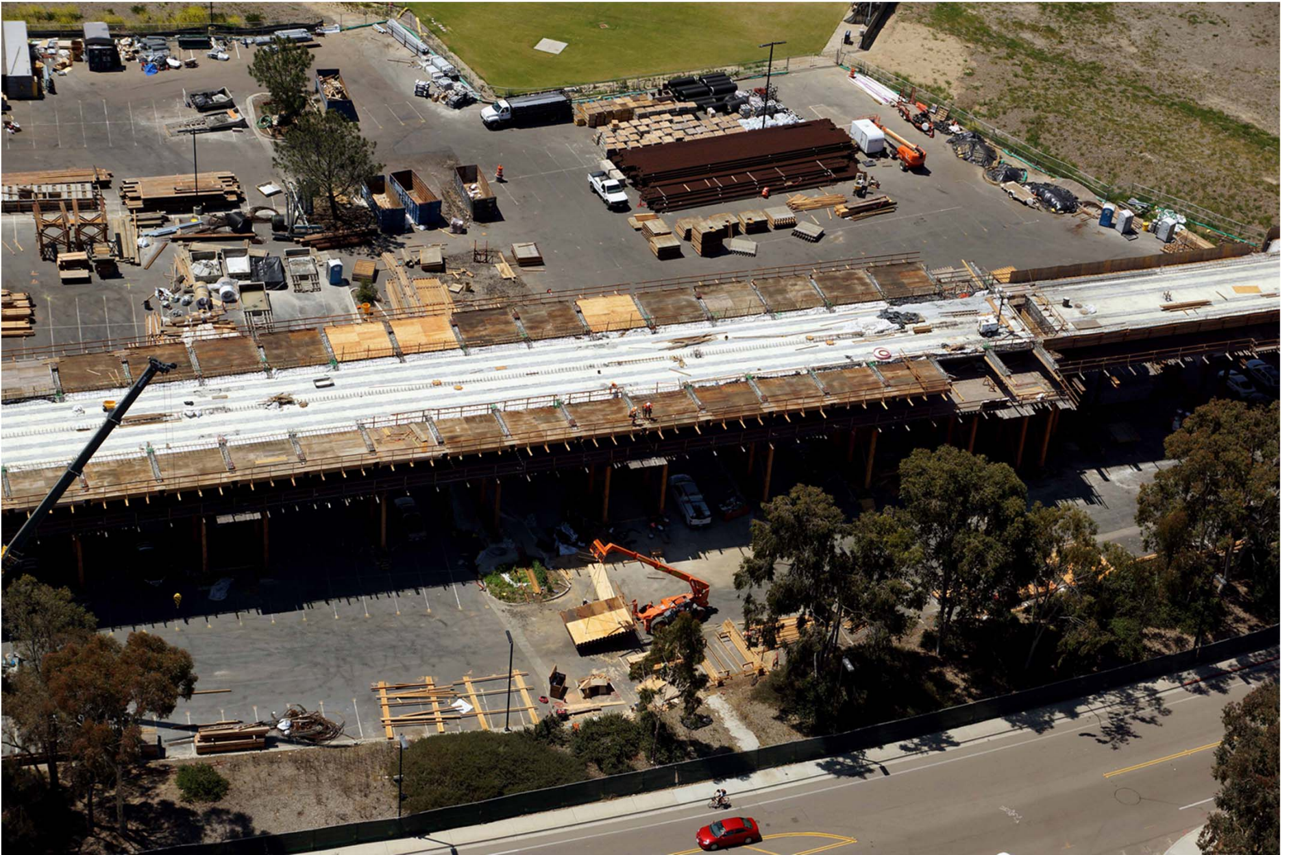
Voigt Drive / UCSD East Station Construction
