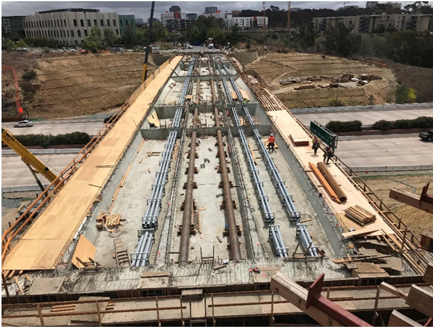
Gilman Bridge, looking east
