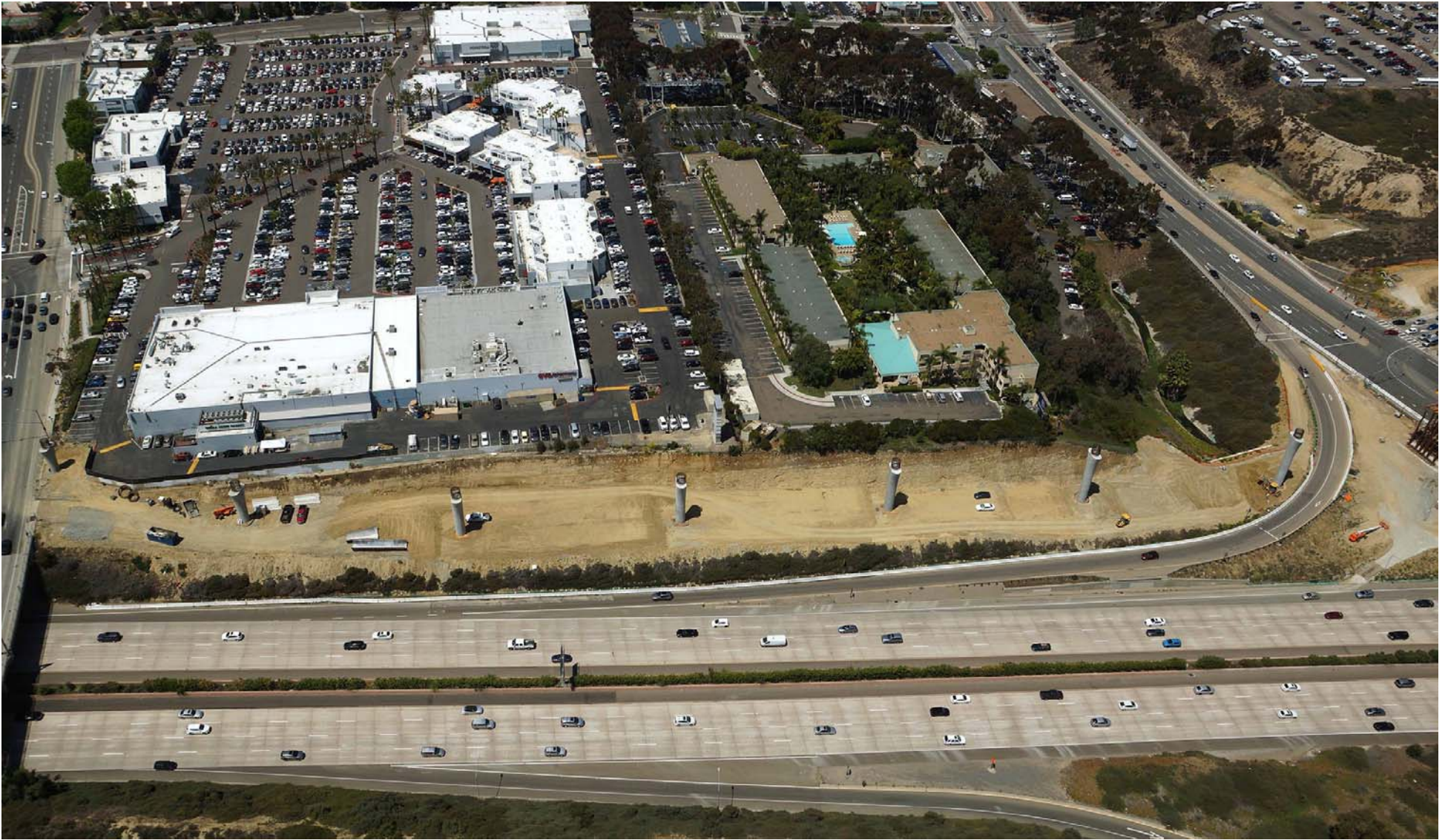
Looking west at Nobel Viaduct progress between Nobel Dr and LJVD
