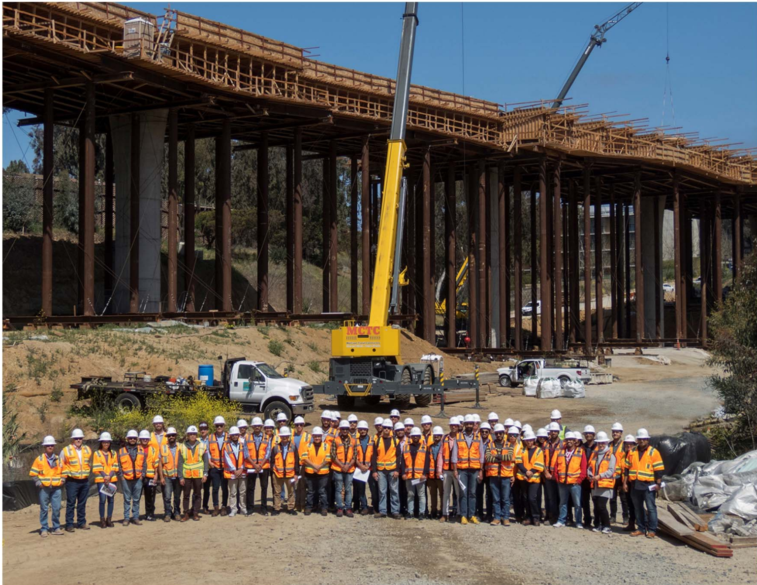
UCSD Viaduct falsework in Pepper Canyon Student Tour
