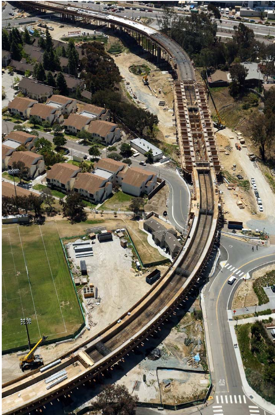
Looking south at Pepper Canyon Station and UCSD Viaduct
