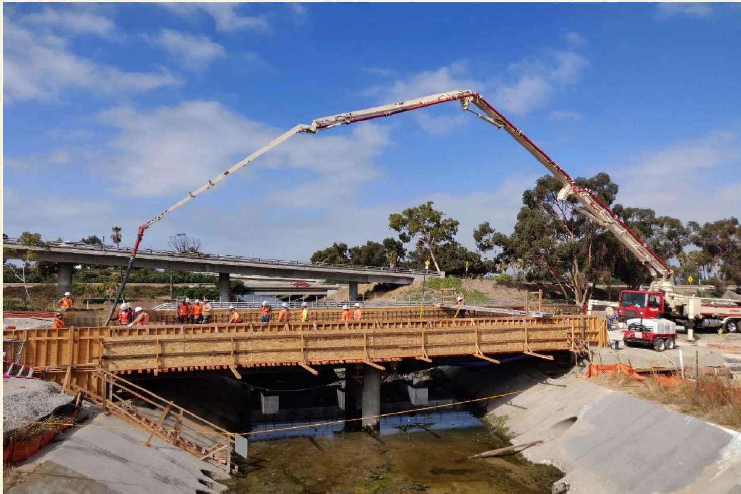
Tecolote Road Trolley Station
