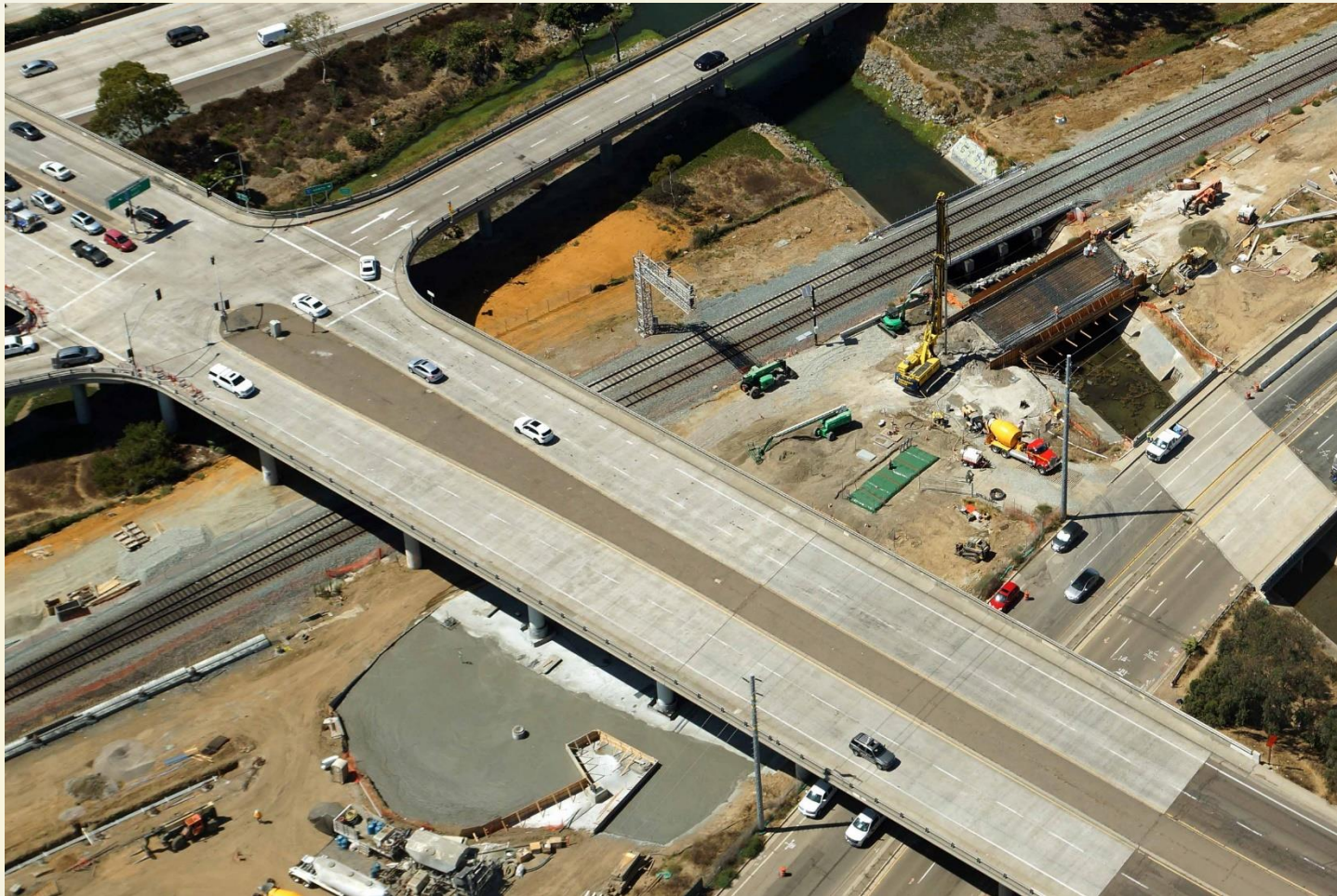
Tecolote Road Trolley Station
