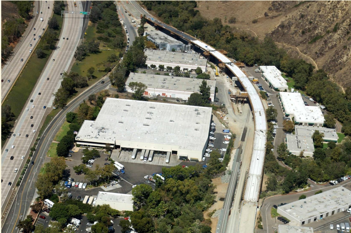
Trolley Flyover along Rose Canyon
