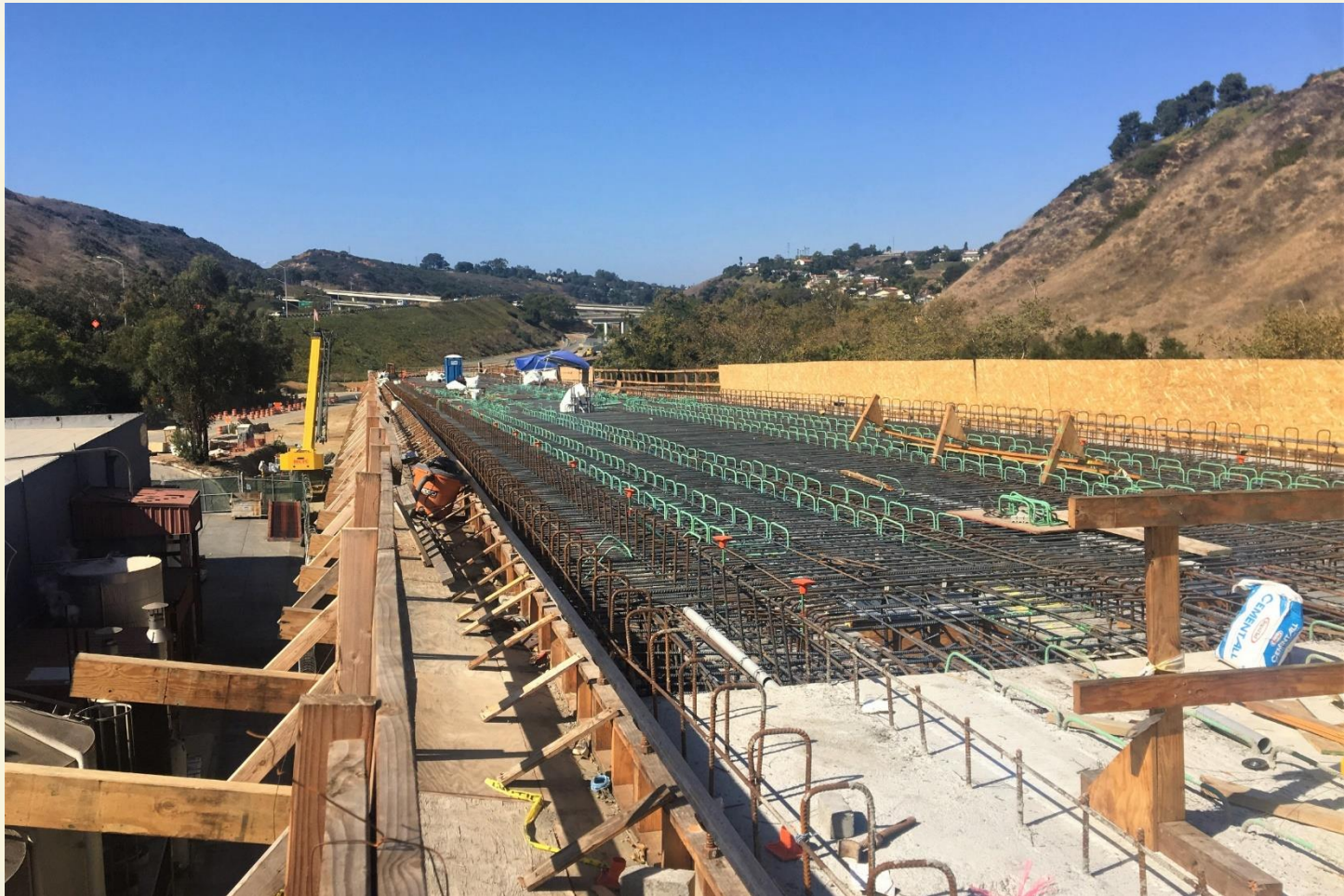
Trolley Flyover along Rose Canyon
