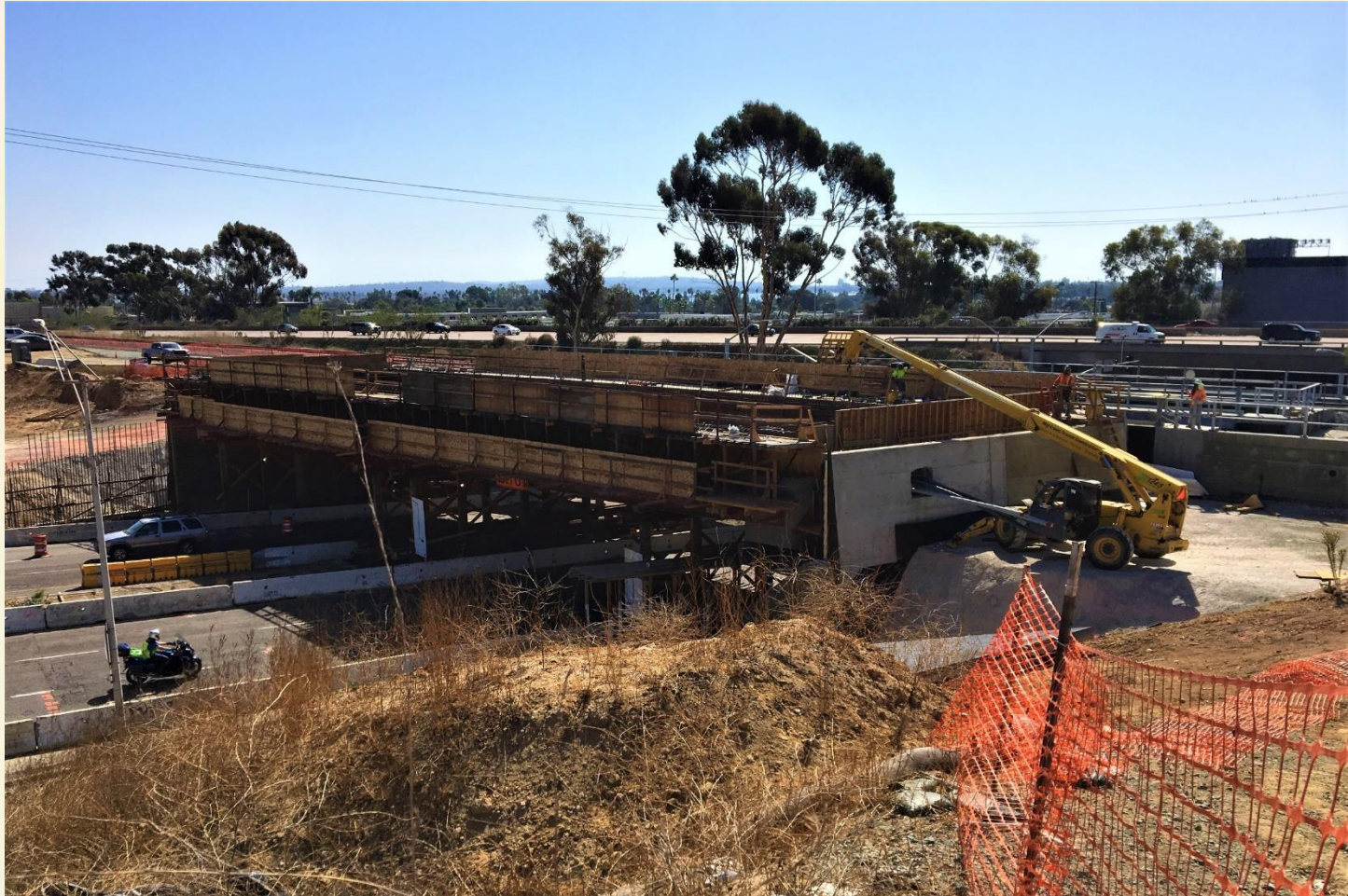
Balboa Avenue Trolley Station
