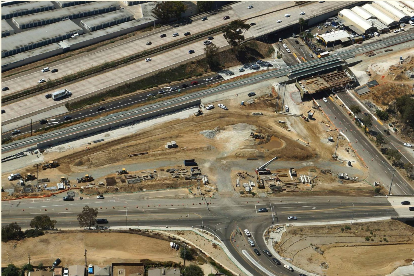
Balboa Avenue Trolley Station
