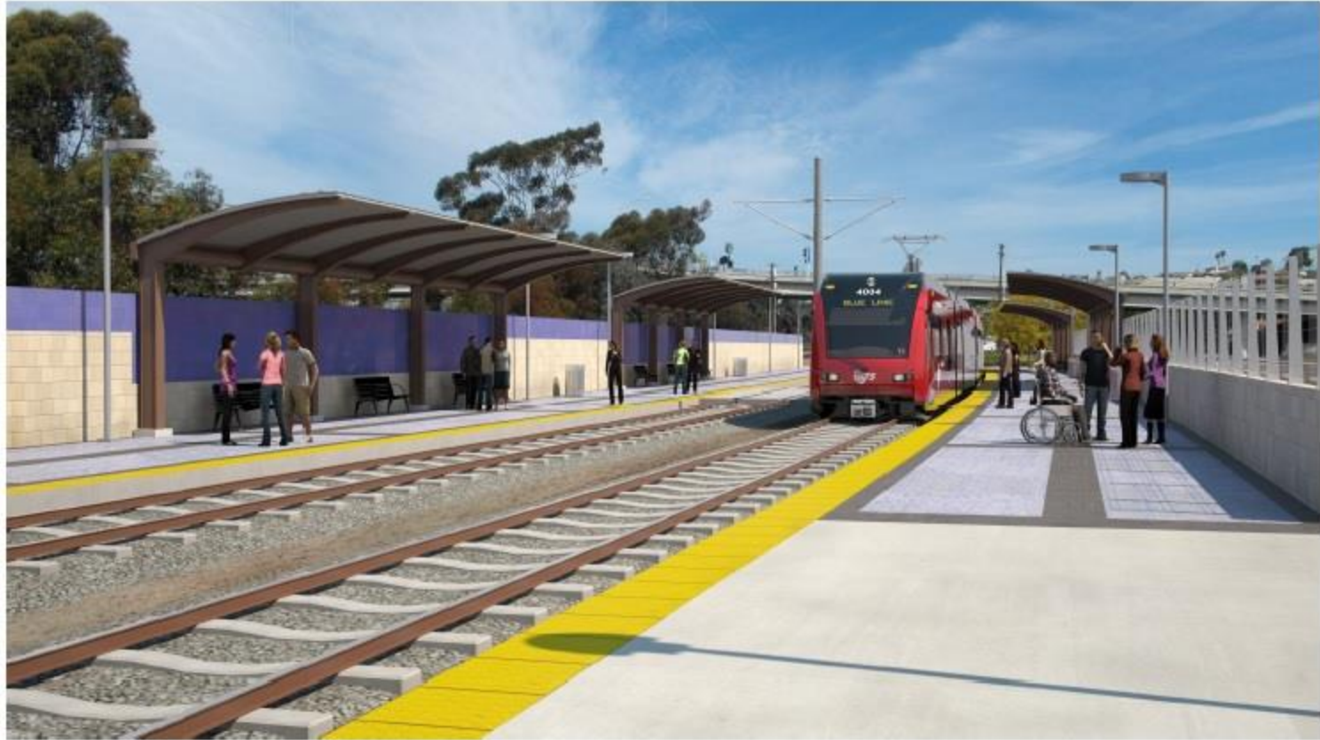
Clairemont Drive Station
