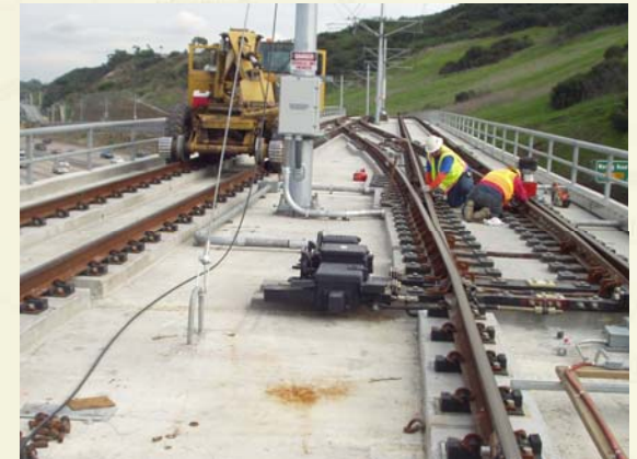
Track work and systems
