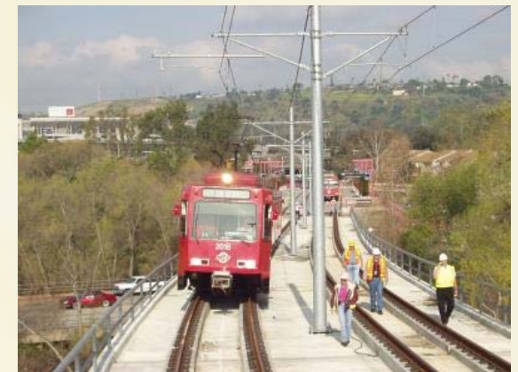
Start-up and testing
