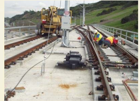
Track work and systems
