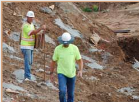
SR 76 project team prepares dynamite cables for bedrock blasting.
