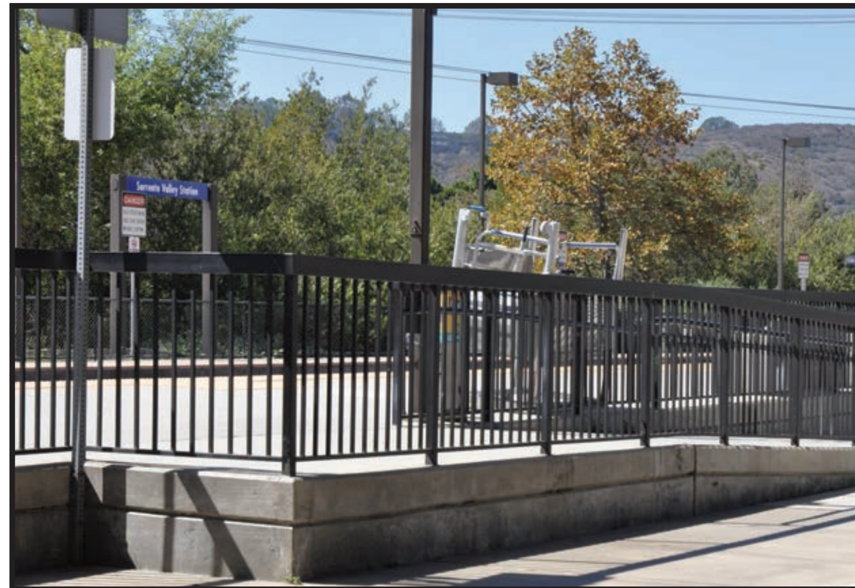
Sorrento Valley Station
