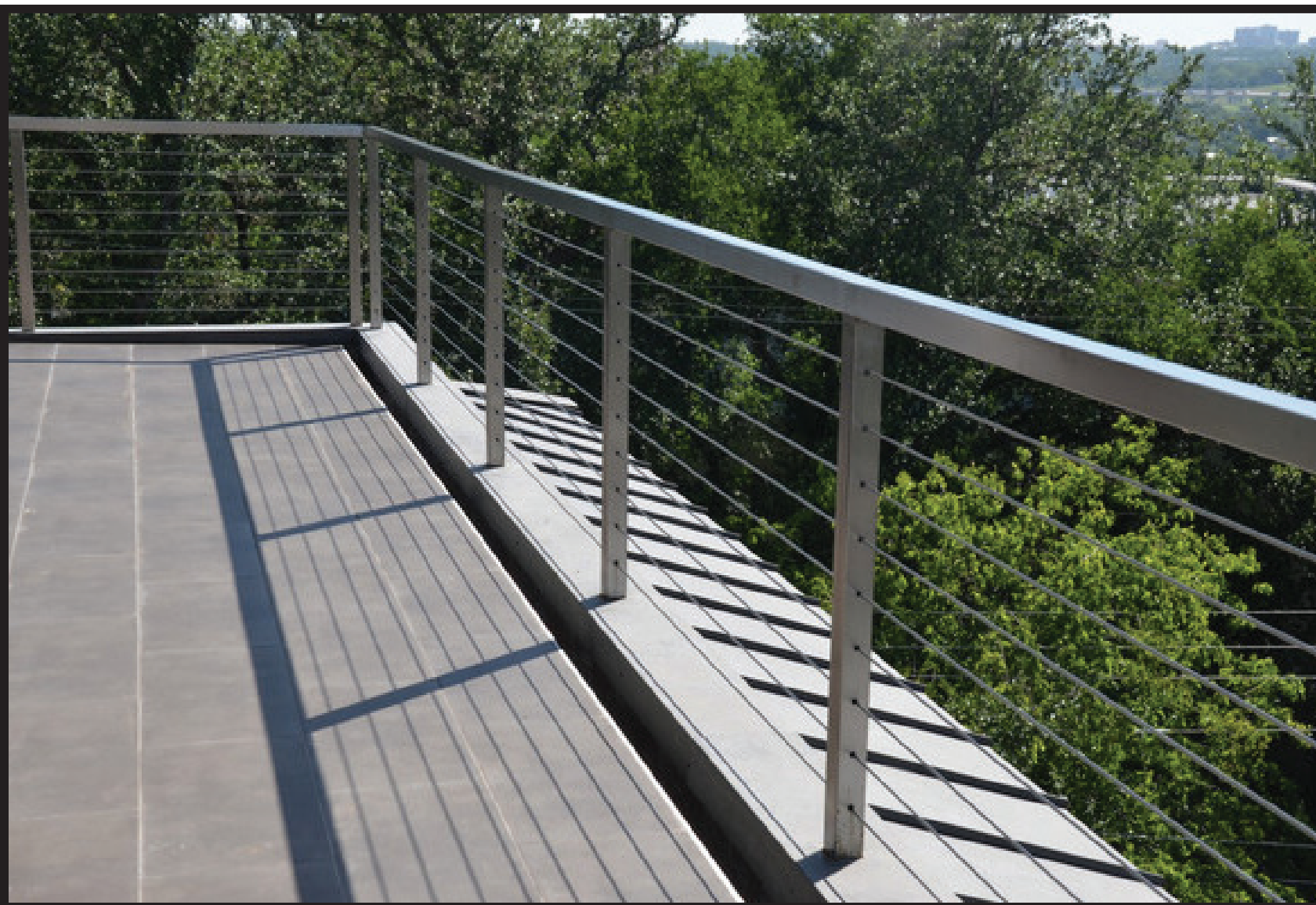
Stainless Steel Post and Cable Railing
