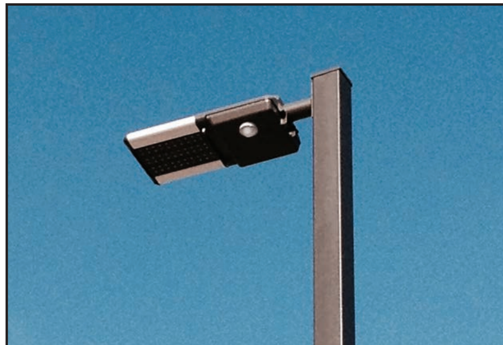
Sorrento Valley Station
