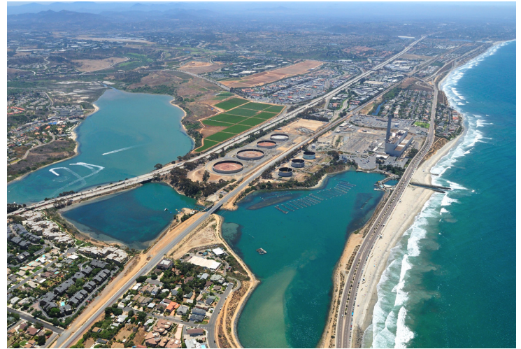
Interstate 5 in the North County traverses six coastal lagoons including the Agua Hedionda Lagoon shown above.
