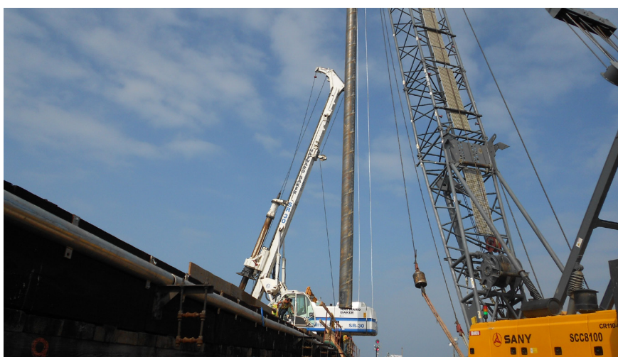
Installation has begun of pre-drilled Cast-in-Steel-Shell piles on the northernmost bridge.
