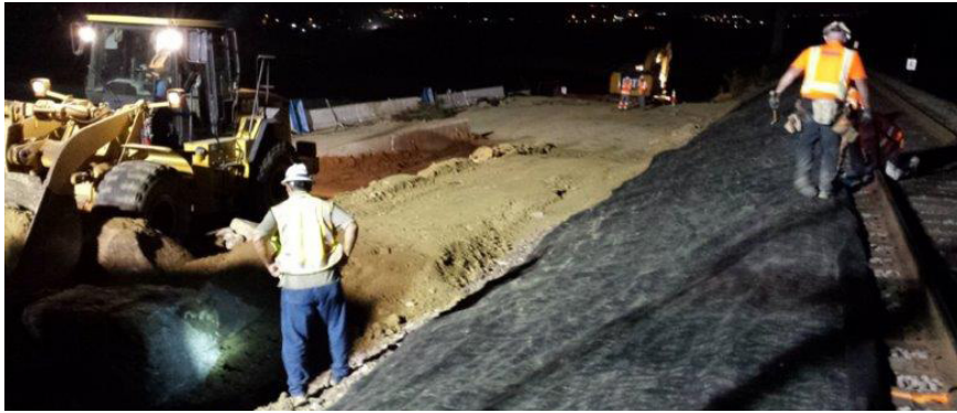
Placing temporary fill and building a support structure.
