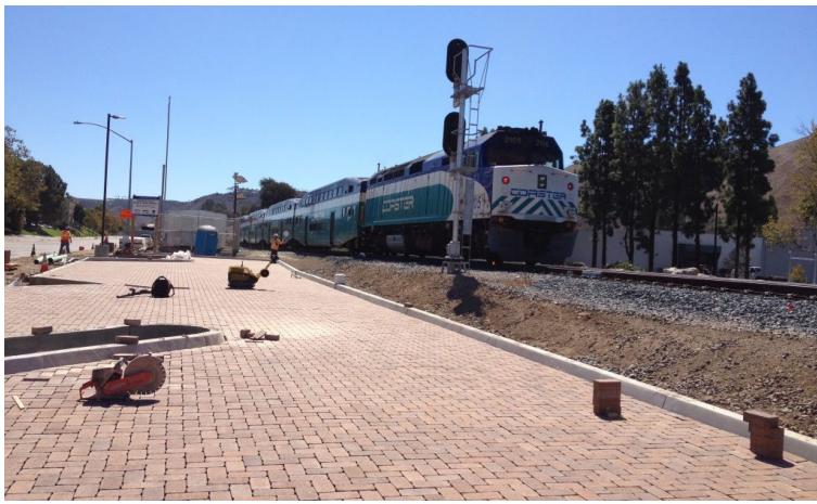
Crews install pavers in the new South Lot.
