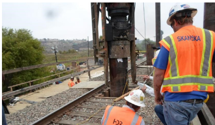
Crews test piles at a mid-lagoon bridge.
