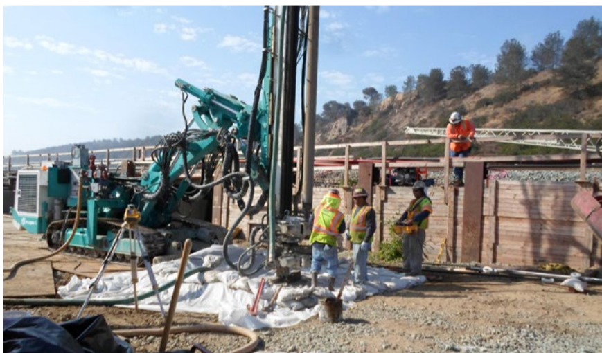
Crews place test piles at a mid-lagoon bridge.
