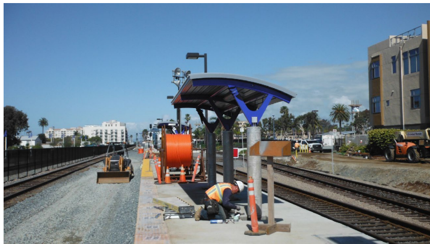
Crews install canopy shelters on the new platform.
