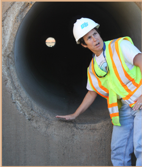
Rush Abrams shows a recently completed wildlife crossing in the SR 76 Middle Segment.
