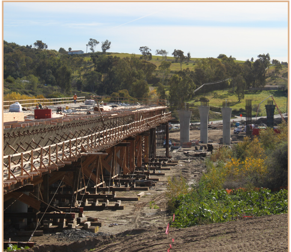
View of San Luis Rey River Bridge construction progress.
