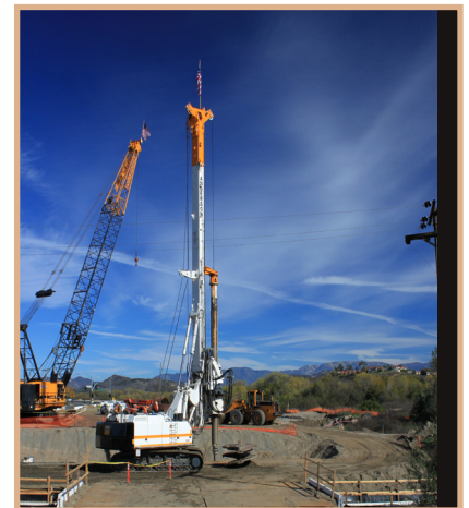
Drilling equipment used to construct Ostrich Farm Creek Bridge.
