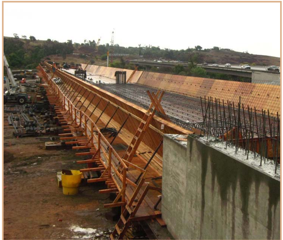
Falsework on the San Luis Rey Bridge
