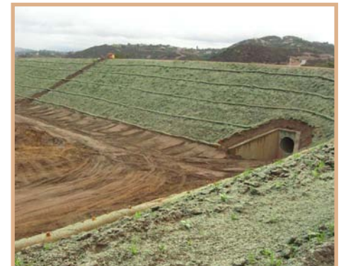
Temporary green emulsion cover & fiber rolls at construction areas
