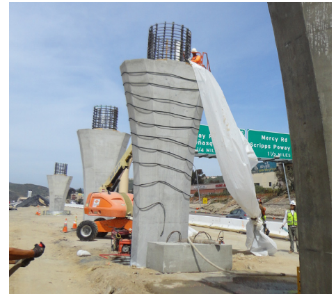
April 2013 - Crews constructing columns that will support the DAR over I-15 in Mira Mesa.
