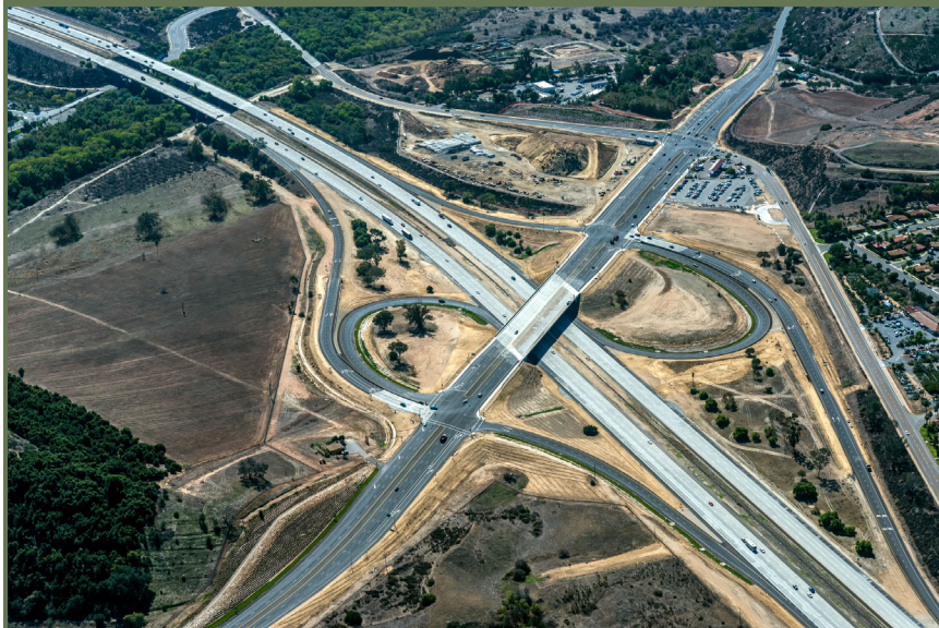
An aerial view looking at the completed SR 76 / I-15 interchange
