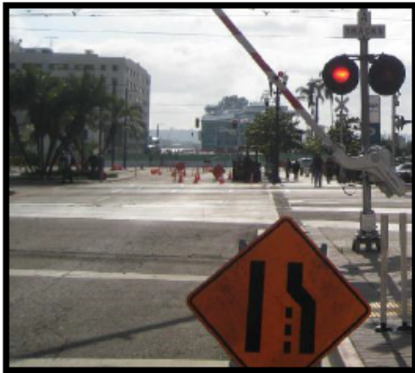
Improper TTC at Broadway railroad crossing, May 9, 2013
