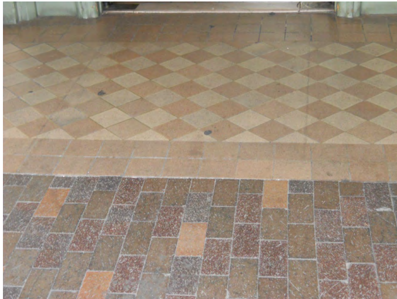
Underneath canopy, historic tile (background) to remain. Brick pavers (foreground) to be replaced with salvaged klinker bricks.
